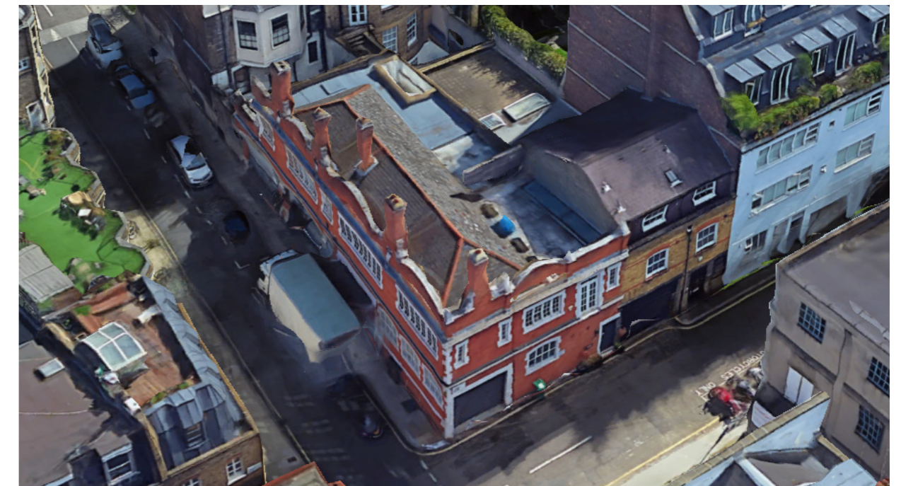
Aerial view of rooftop to 25 John's Mews.
