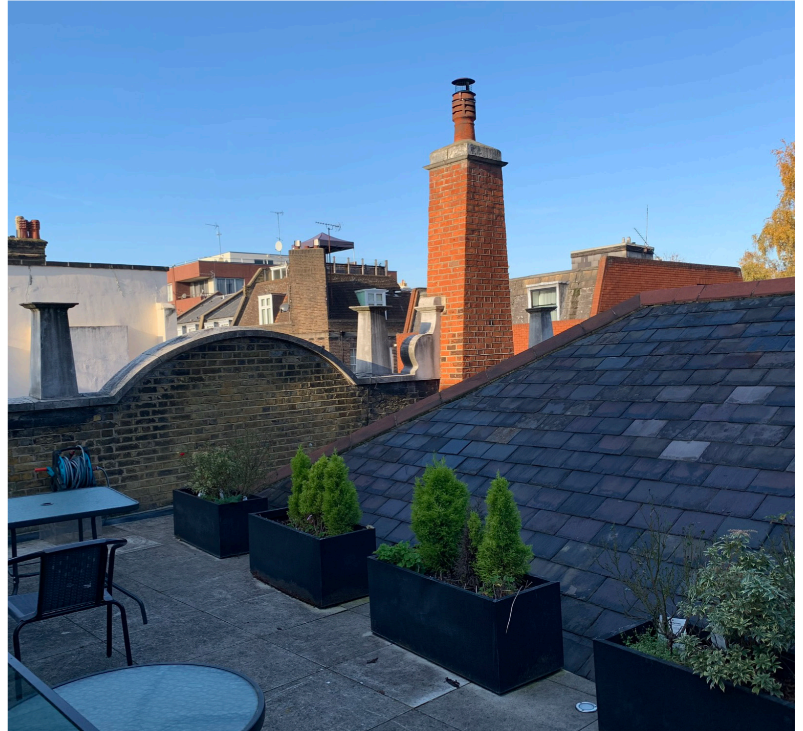
A photograph taken on the 01/08/2022 showing the existing slate roof.
