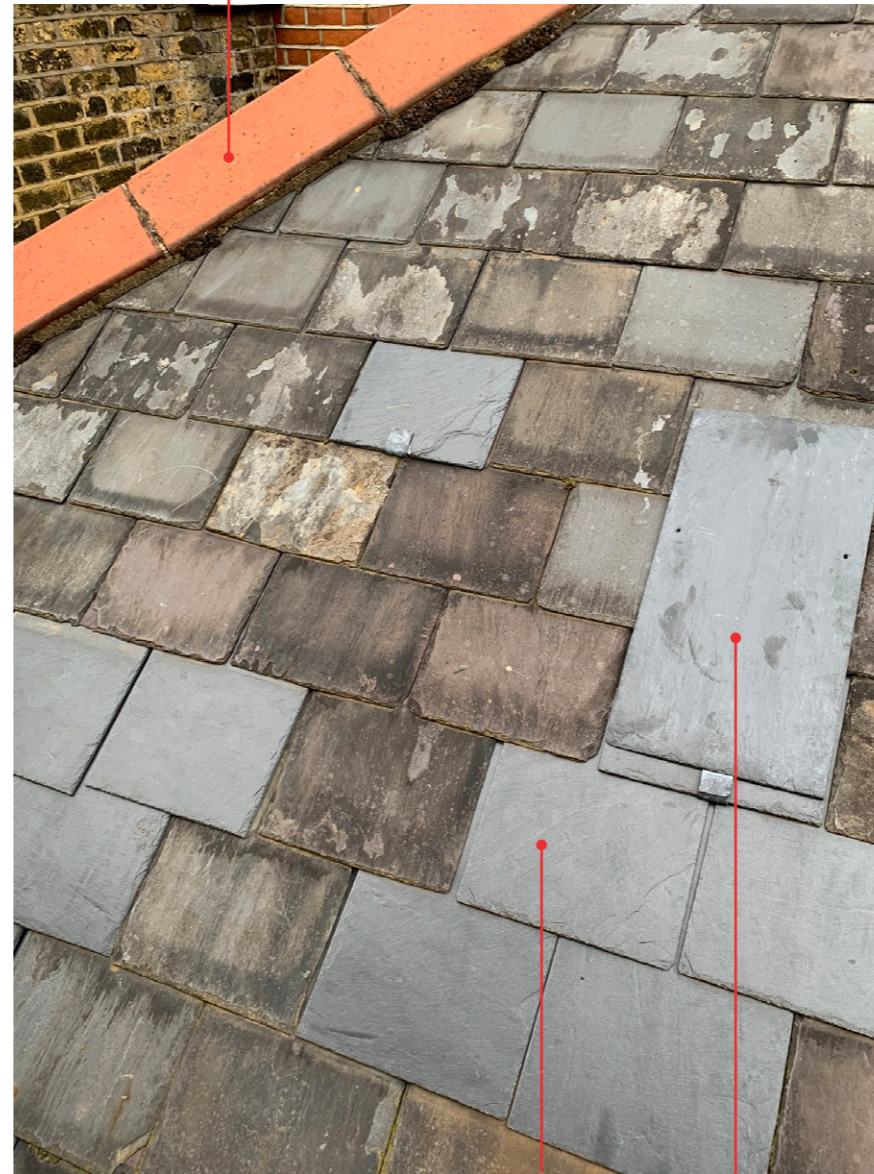
Existing slate roof.
