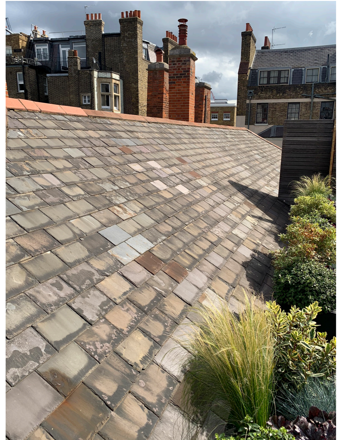
A photograph of existing slate roof taken in August
