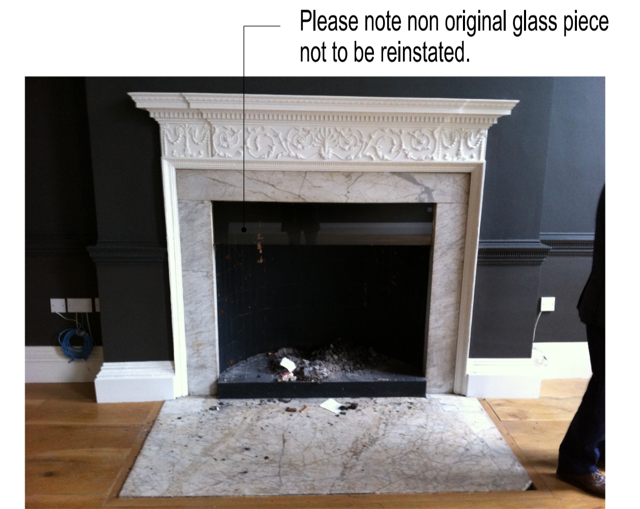
CHIMNEY PIECE IN ONSITE STORAGE TO BE REINSTATED
