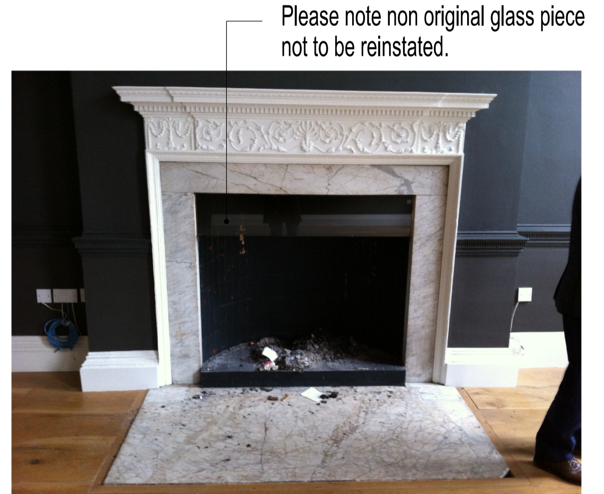
CHIMNEY PIECE IN ONSITE STORAGE TO BE REINSTATED
