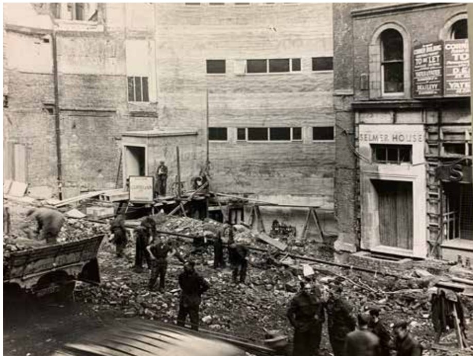
Figure 3.11 1941 bomb damage. The Site is located on the right. Source: Camden Local Archives
