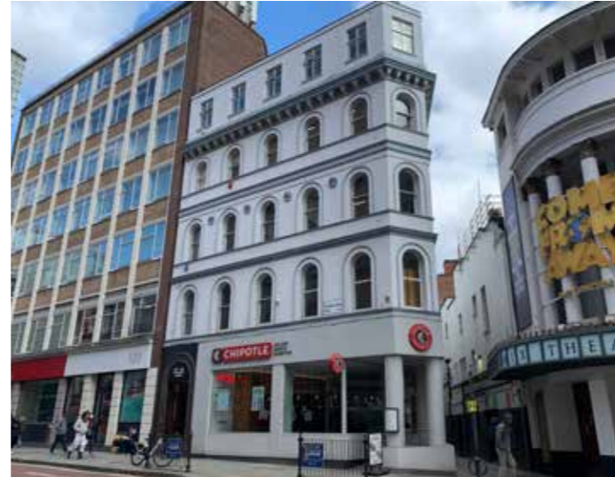
Figure 4.1 Front, west elevation of the Site.
