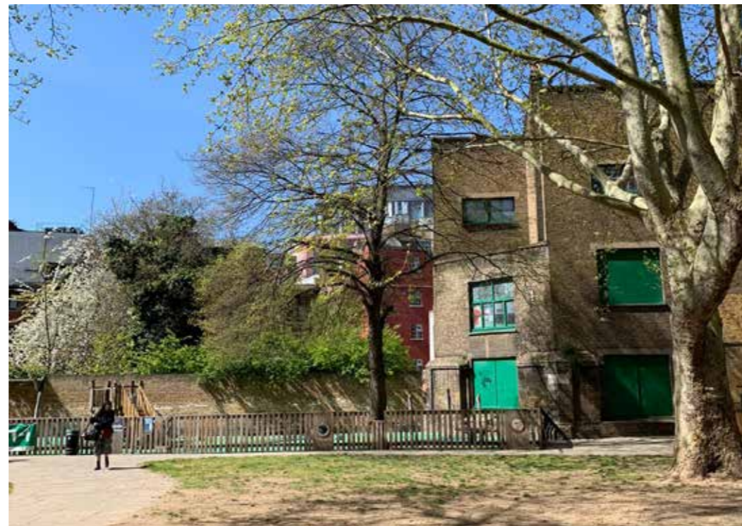
Figure 4.8 The Site is obscured from view from the churchyard of St Giles in the Fields due to the presence of Elms Lester Painting Rooms
