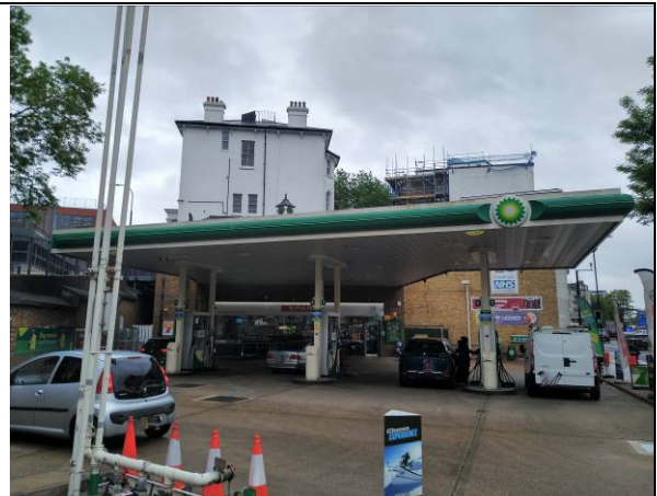
Photograph 2 – View looking east over the garage forecourt showing the extent of the hardstanding on site.
