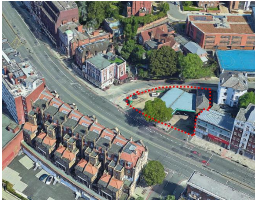
Figure 1 - Aerial photo of the Site and neighbouring buildings (© Google)
