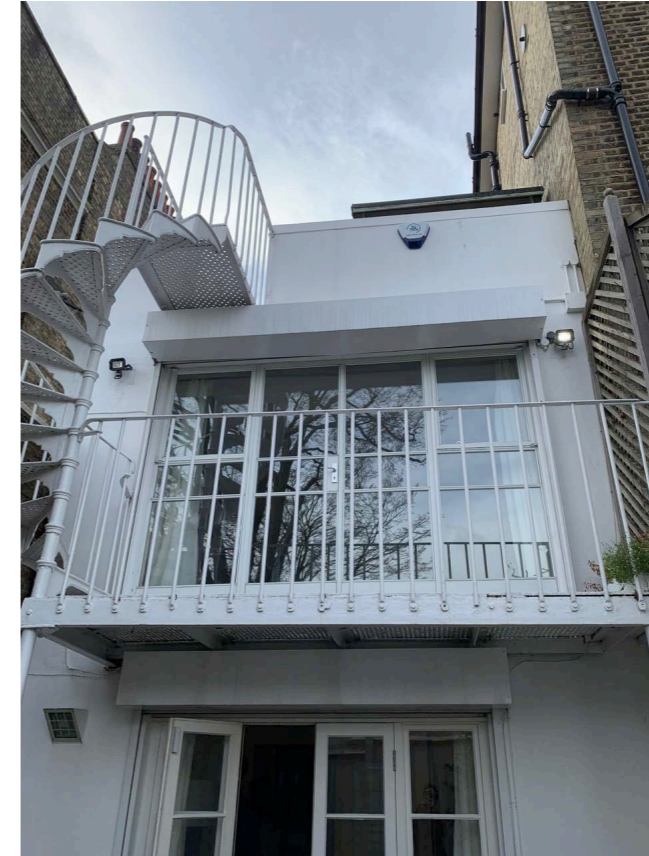
4. Rear of No.4B Upper
