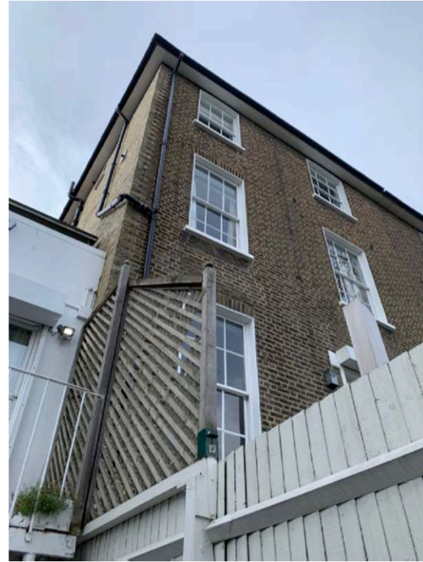
2. Rear of No.4B Looking up at No.4
