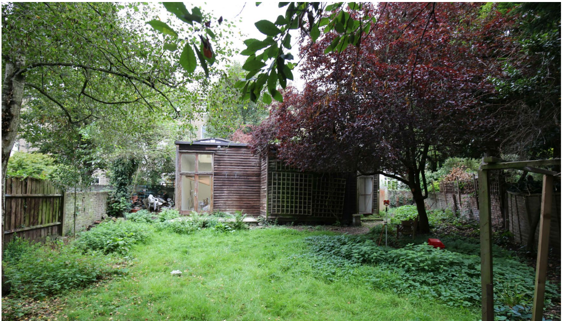
Fig. 2: View of Existing south-east elevation of Artist's Studio (photo courtesy of LBMV Architects)
