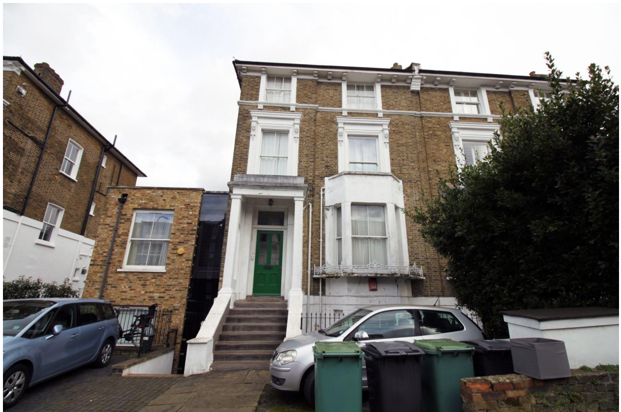
Fig 5 : Front elevation of 2 storey 42D maisonette (left) & 4 storey main house at 42 Parkhill Road
