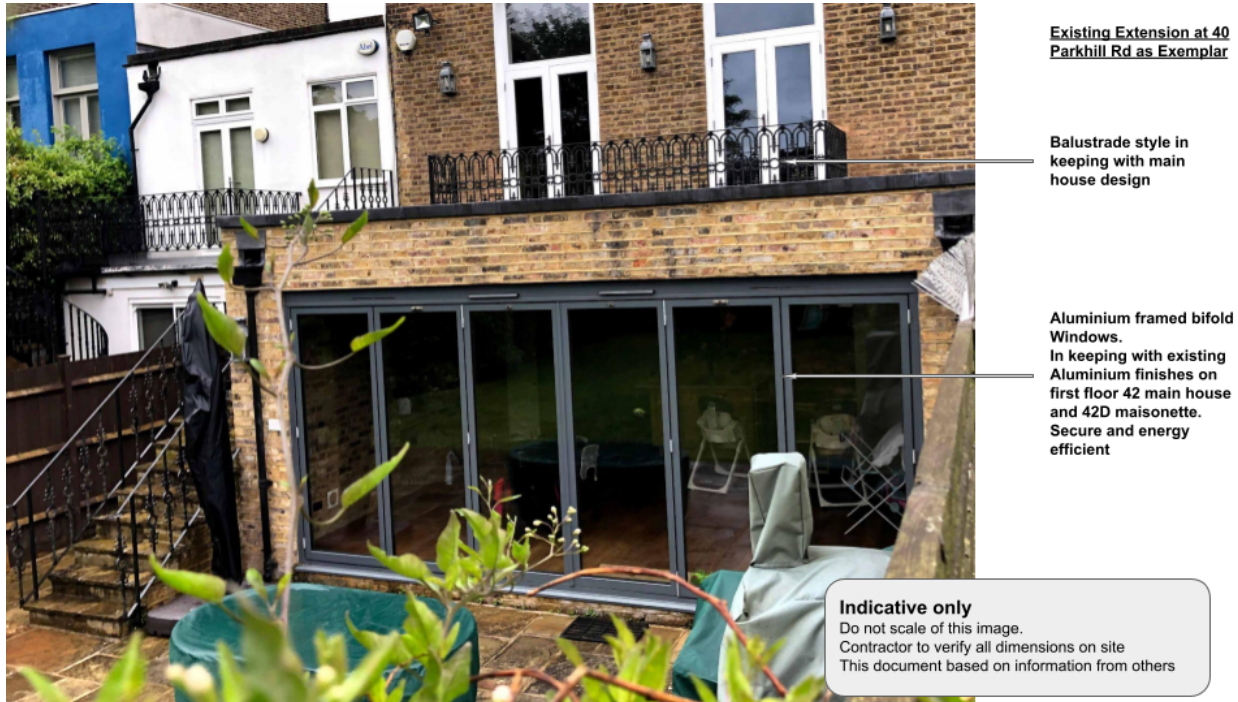
Fig 10 : Existing rear extension at adjacent no 40 - illustrating indicative materials for balustrades, aluminium windows and london stock brick in sympathy and character with the main building
