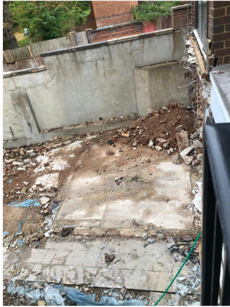
Photograph 6: Demolition of Existing Ground Floor
