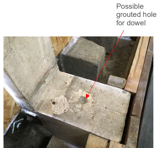
Figure 2.3 – Photo showing possible grouted hole for dowel at fin
