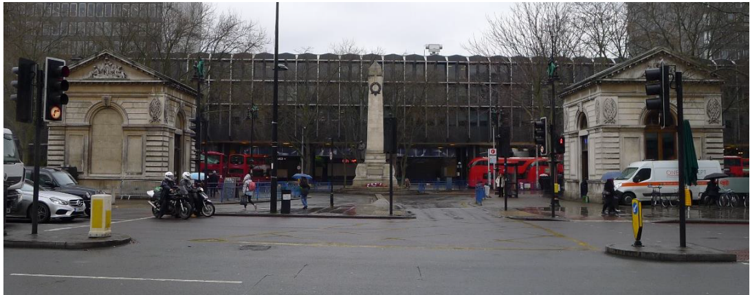
Figure 3: View of the two Lodges flanking Euston Grove and framing the War Memorial
