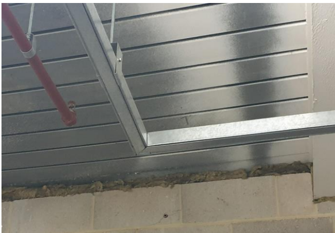
Figure 49 Insulation behind the concrete block wall
