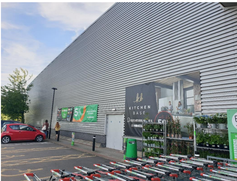
Figure 27 Sandwich panels
