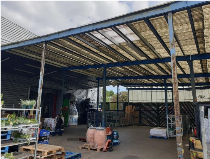
Figure 18 Service yard entrance canopy and service yard area canopy
