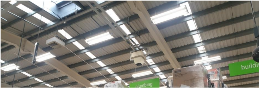
Figure 42 Main building roof – polycarbonate panels
