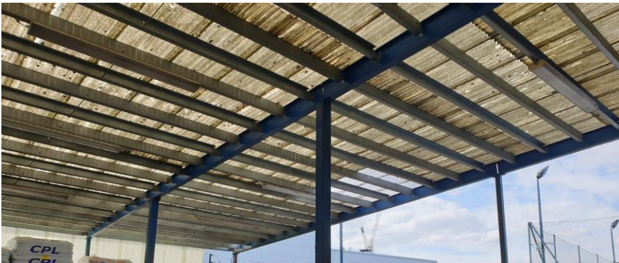
Figure 44 Service yard roofing – GRP panels
