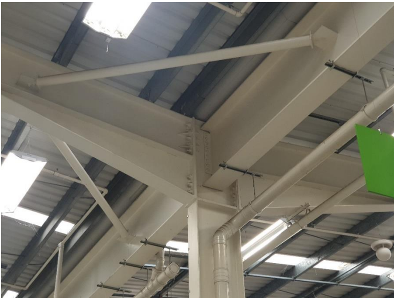
Figure 16 Typical detail of a primary frame
