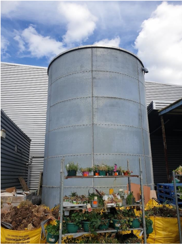
Figure 23 Sprinkler tank
