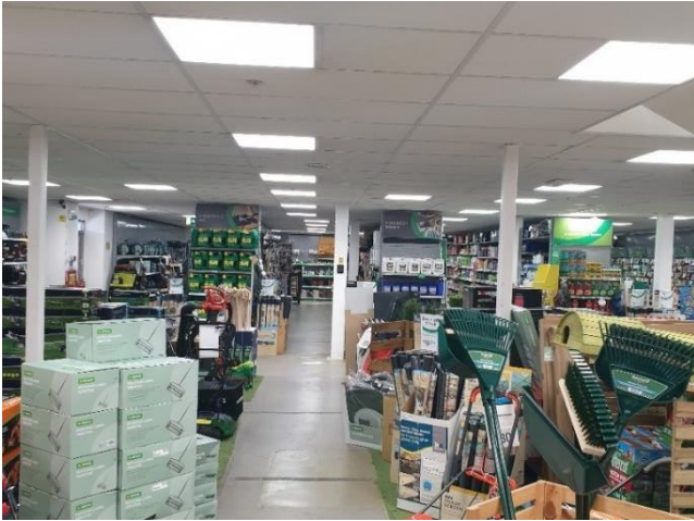
Figure 52 Mezzanine – sales area WEEE lights (approximately 175 units)
