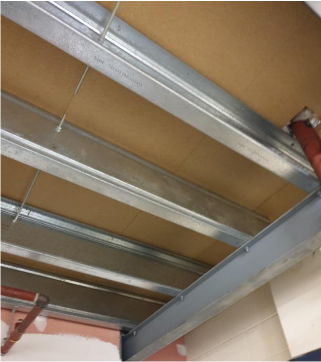
Figure 34 Timber-based panels on mezzanine floors
