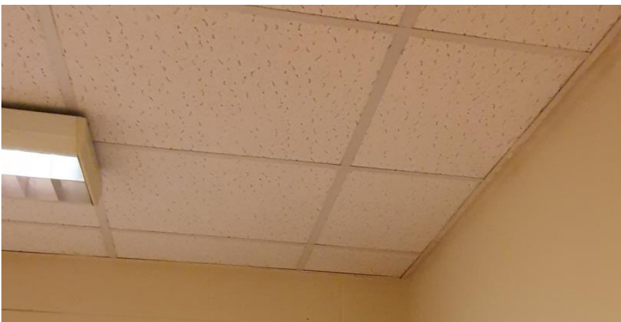
Figure 45 Staff areas and entrance lobby ceilings – polystyrene ceiling tiles
