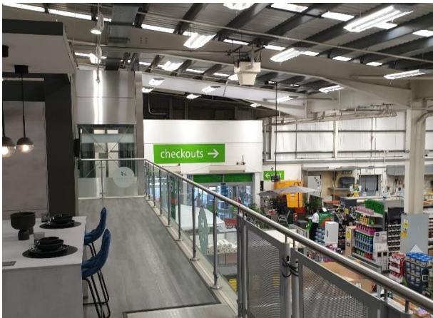
Figure 38 Sales mezzanine – glazed balustrades
