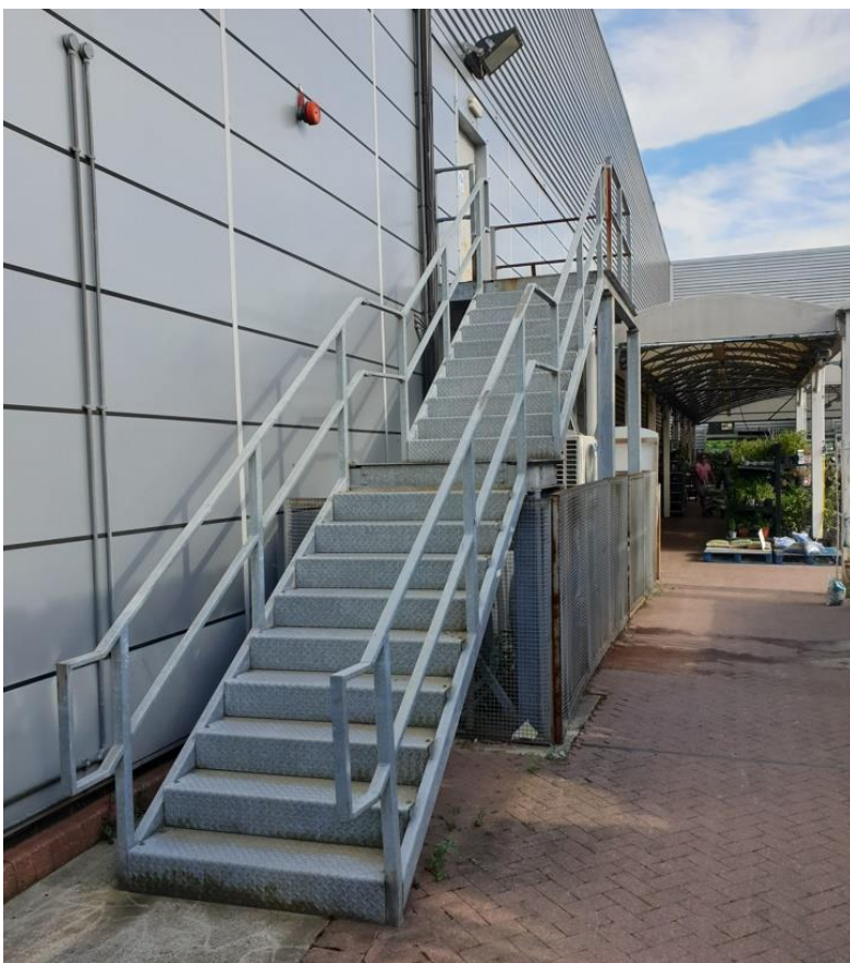
Figure 26 External stairs (fire exit) near the flower garden
