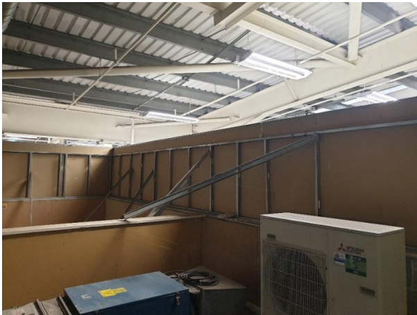
Figure 32 Timber-based panels covering the plant room
