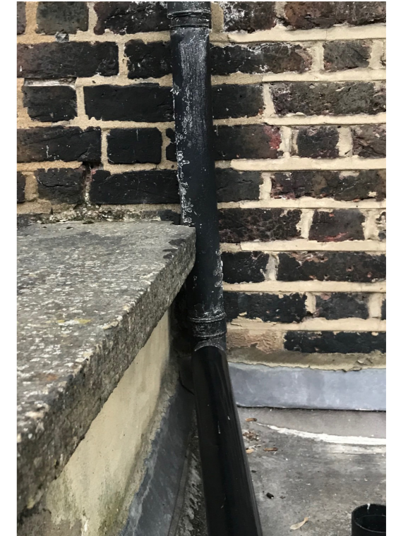
Figure 2H Junction between existing rainwater goods + modern PVC addition
