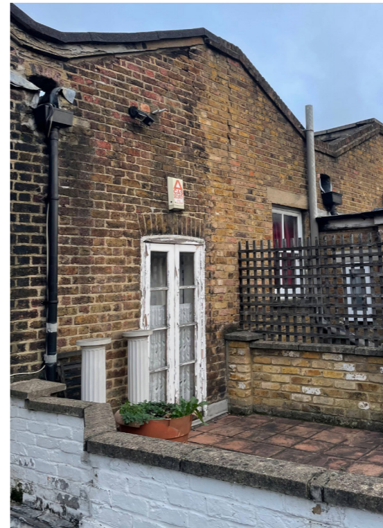
Figure 3H Existing masonry wall to terrace of no.21 Kelly Street
