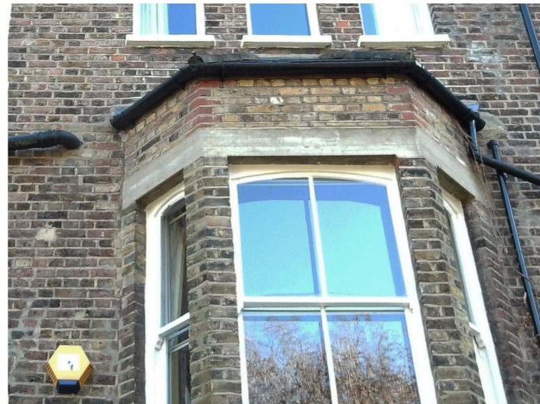
d) view of existing bay window with concrete lintel
