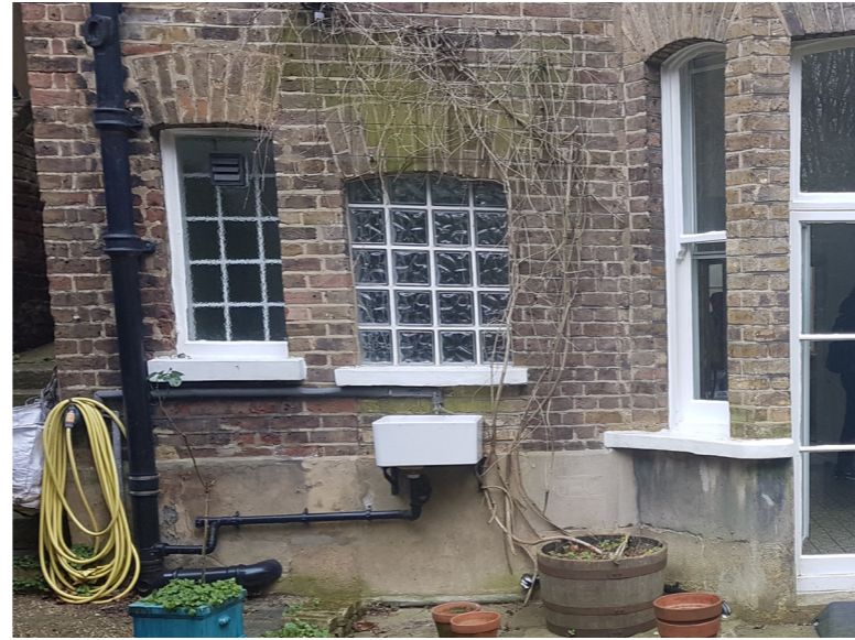
e) view of existing LGF rear windows on exposed concrete footings
