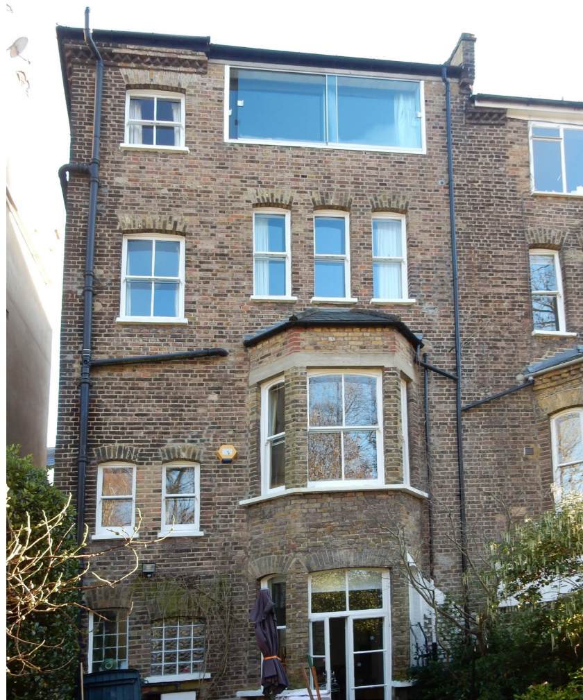
c) view of existing rear elevation of house
