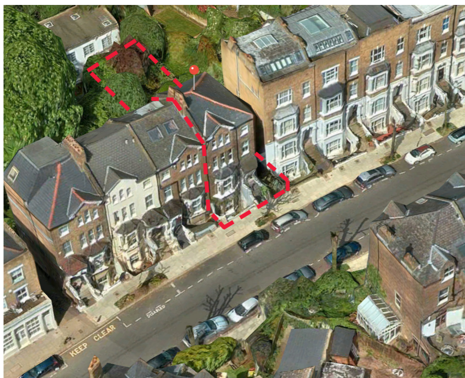
a) Aerial view of 22 South Hill Park from front showing front areaway
