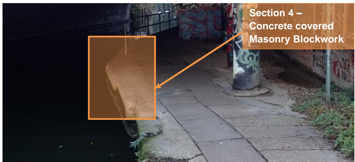
Figure 3.70: Photograph indicating Section 4 - Concrete covered Masonry Blockwork Wall
