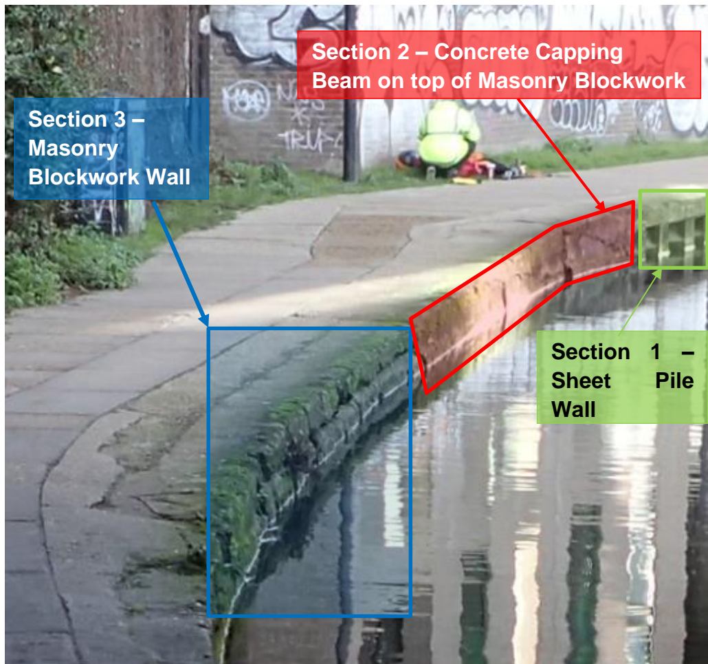
Figure 3.3: Photograph indicating Wall Section 1,2 & 3
