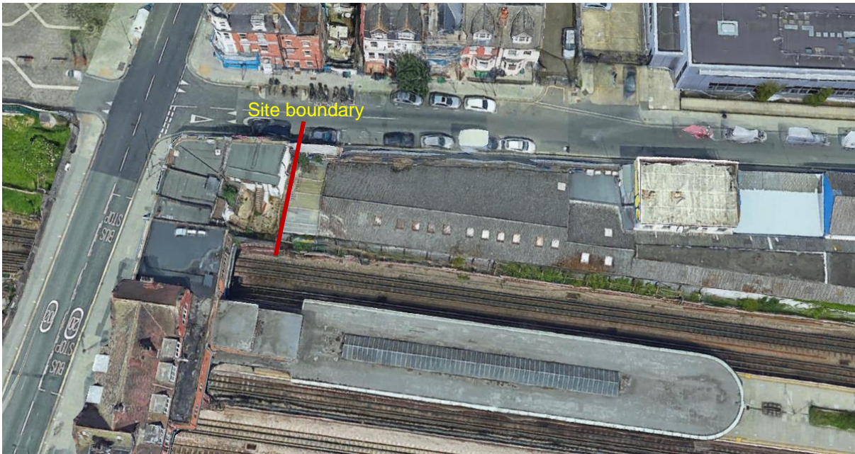
Figure 5 Adjacent infrastructure to plot S8
