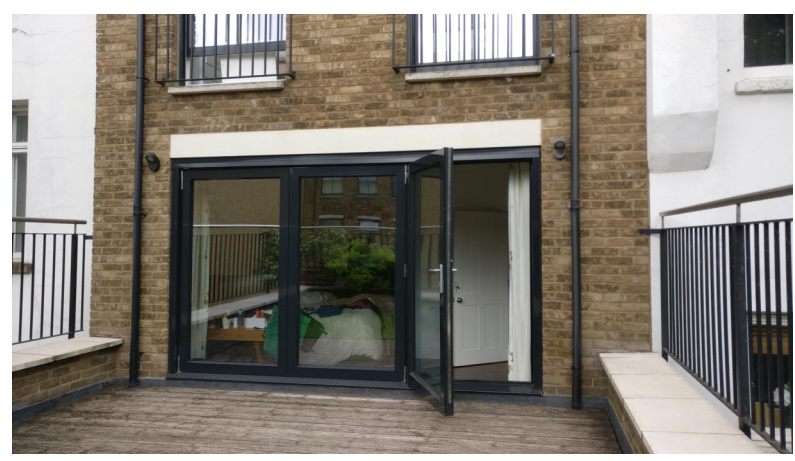
IMAGE OF EXISTING DOORS
