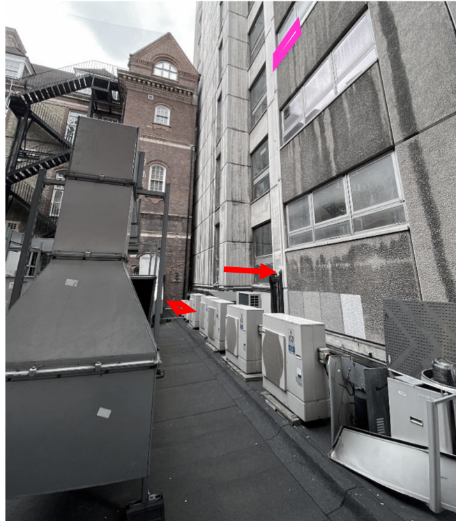
Photo overlay indicating proposed condenser unit (red) and medical gas pipework (magenta) approximate locations
