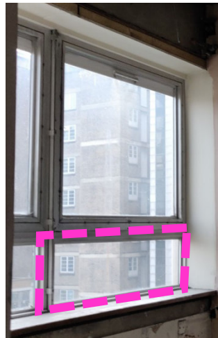
Internal window within third floor within Queen Square House (above) with proposed replacement Perspex panel location dashed
