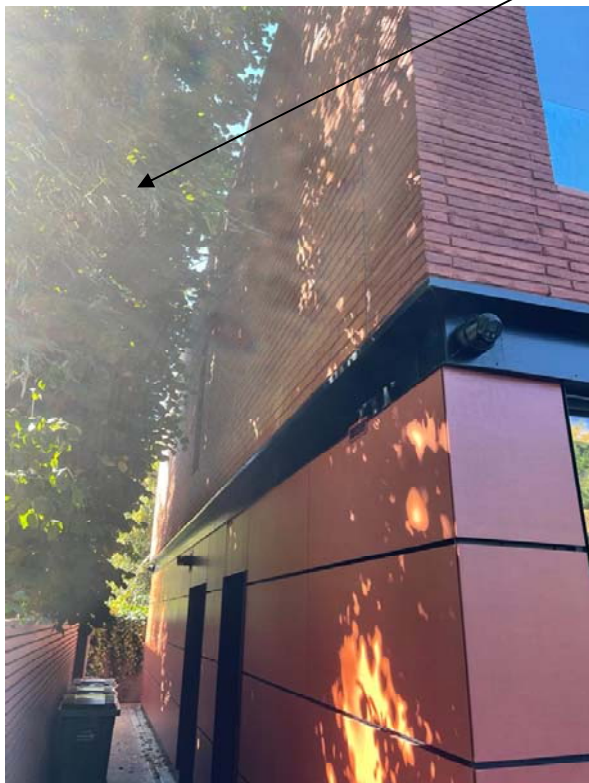
side wall along the boundary
