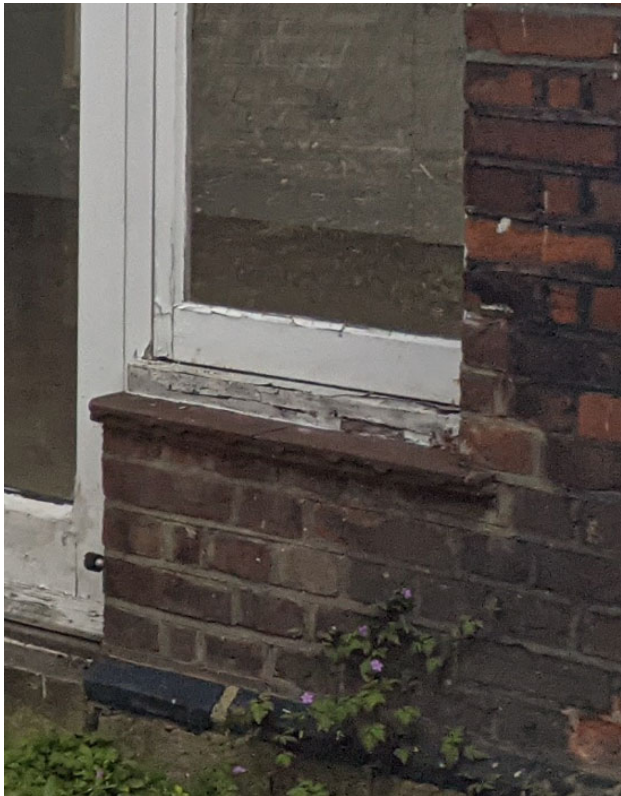
Figure 5. Existing modified brickwork beneath glazed screen, indicating non-original
