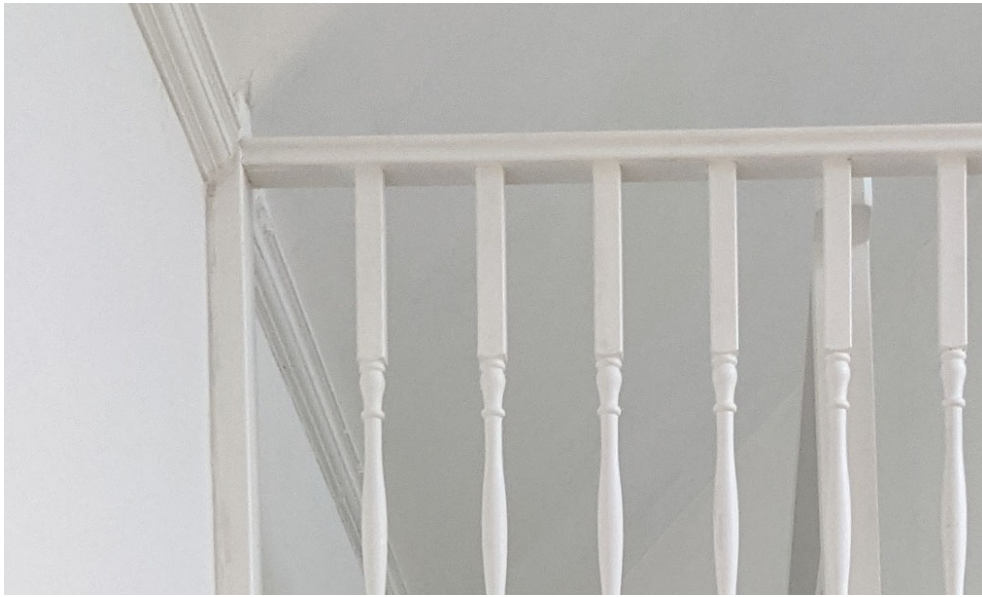
Figure 8. Original timber rail that has been crudely cut to allow for the installation of a mezzanine
