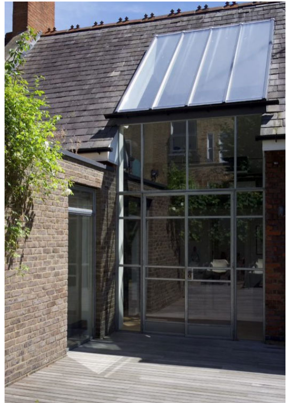
Figure 6. Modern refined glazed screen as installed at 4 Primrose Hill Studios
