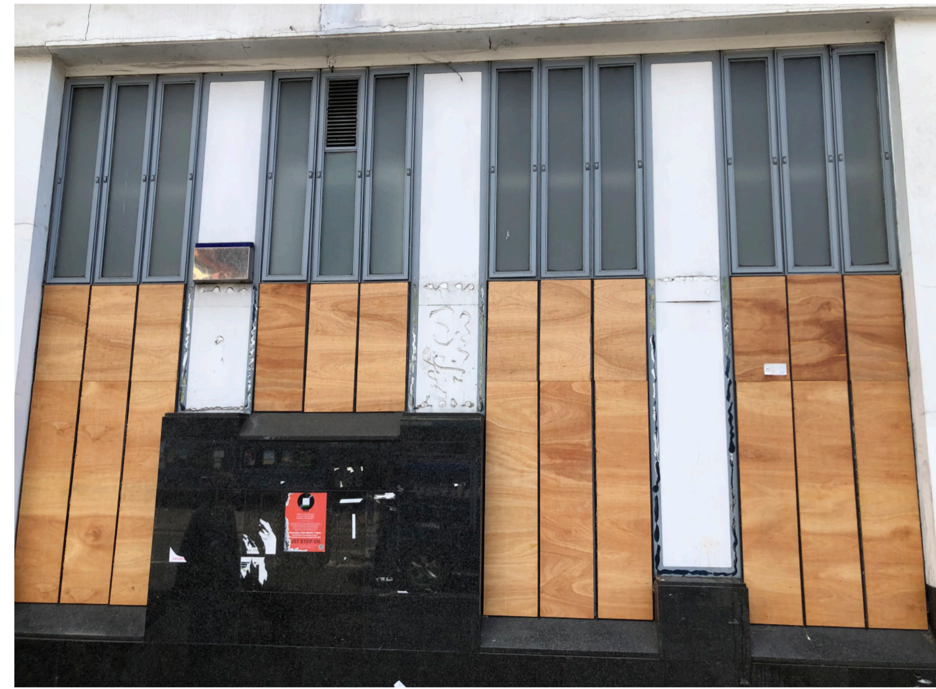
EXISTING (ATM) SURROUND TO BE REMOVED TO REINSTATE ORIGINAL ARCHITECTURE. NEW WINDOWS
