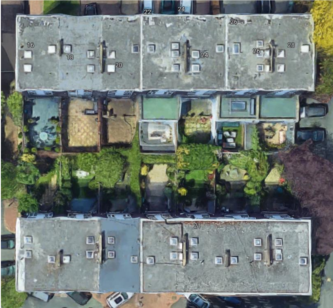
4. Ariel View of rear gardens to properties nos 16-28 (including no. 24 application site), and nos 33-39 Elliott Square
