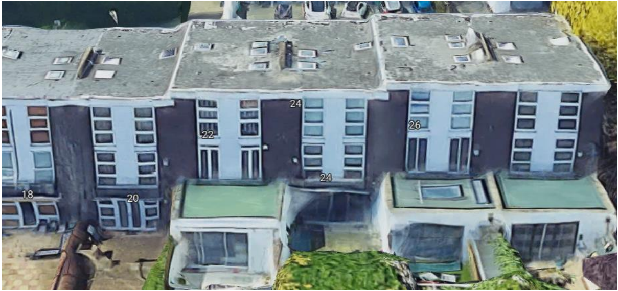
3. Rear elevation of 24 Lower Merton Rise (application site) and rear of terrace nos 18-28 (even)
