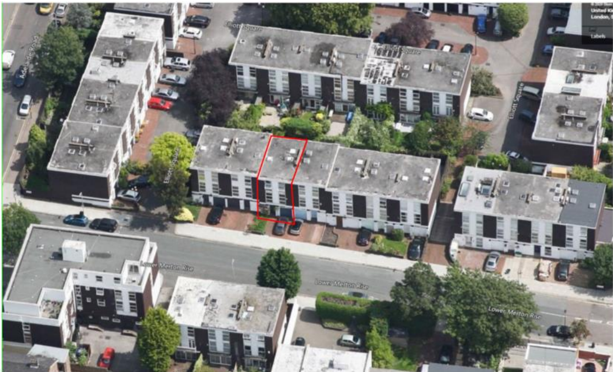
2. Ariel View of 24 Lower Merton Rise within terrace nos. 16-28 (even)
