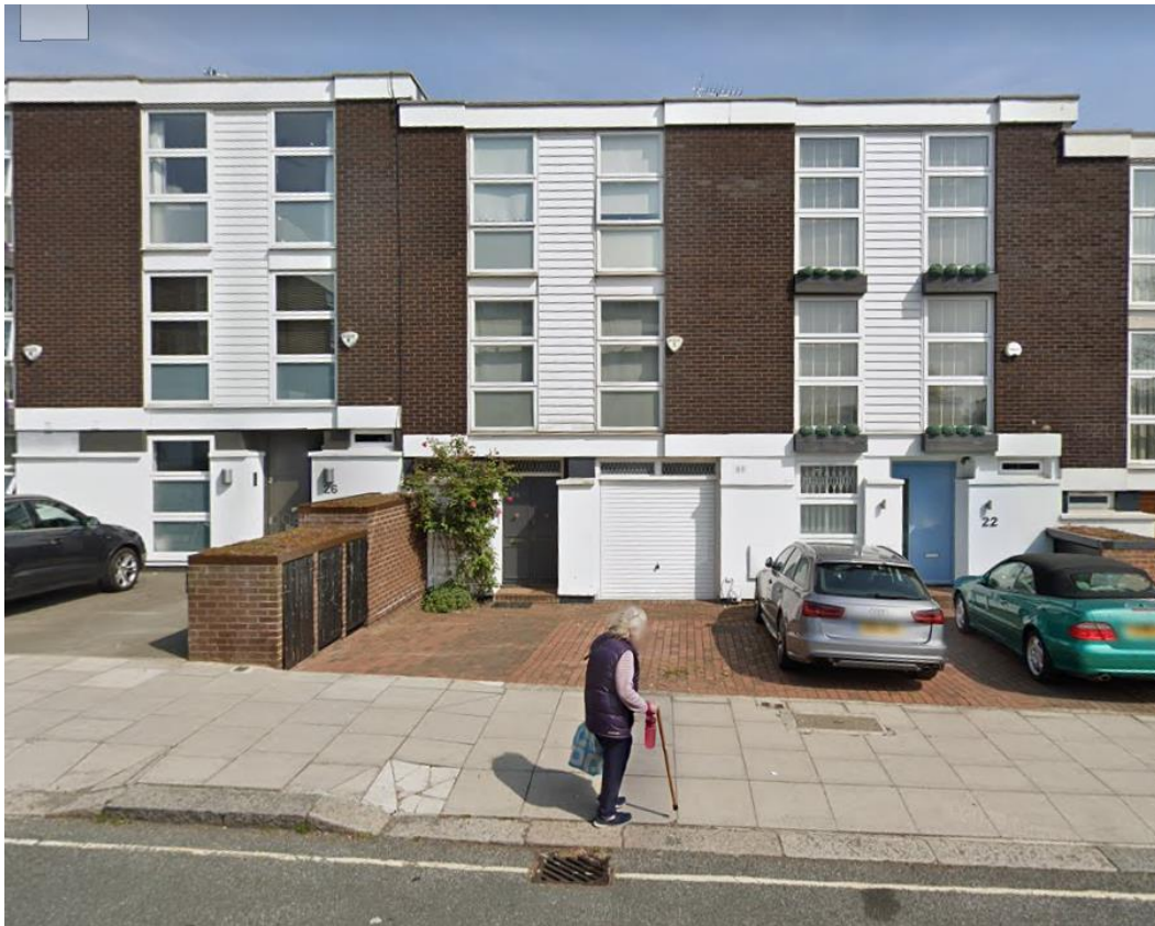
1. Front elevation of 24 Lower Merton Rise in centre (application site), no. 26 to the left and no. 22 to the right
