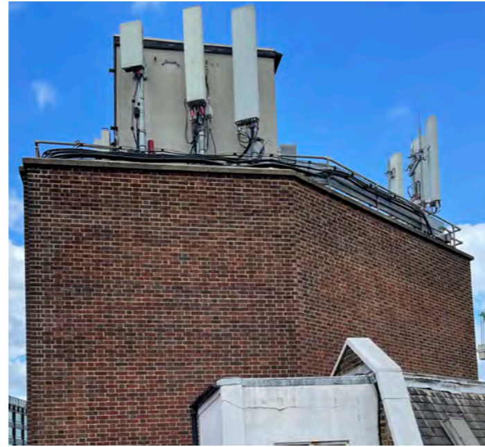
north towards no. 120 plant room and mobile antennas
