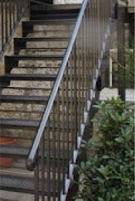
Reference image: Wrought iron traditional external staircase
