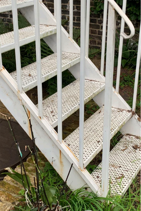
Existing white metal staircase
