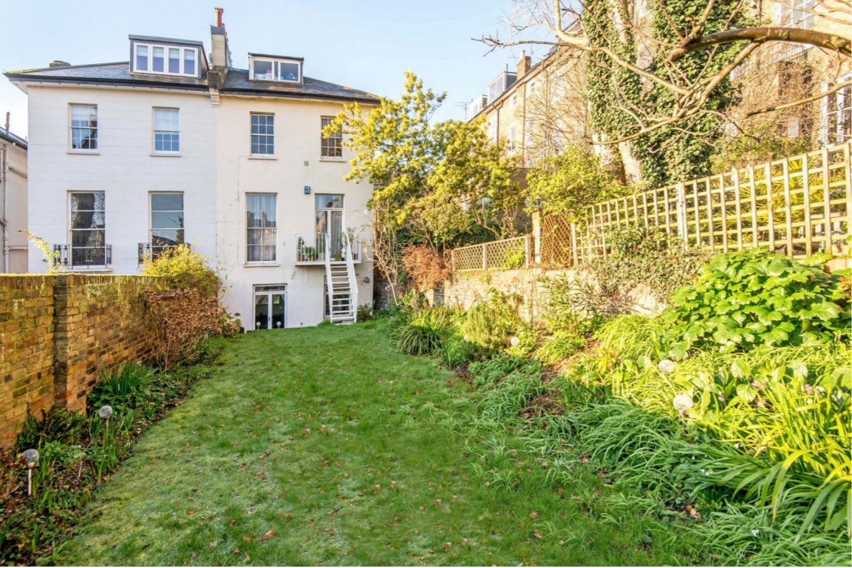
Existing rear facade
