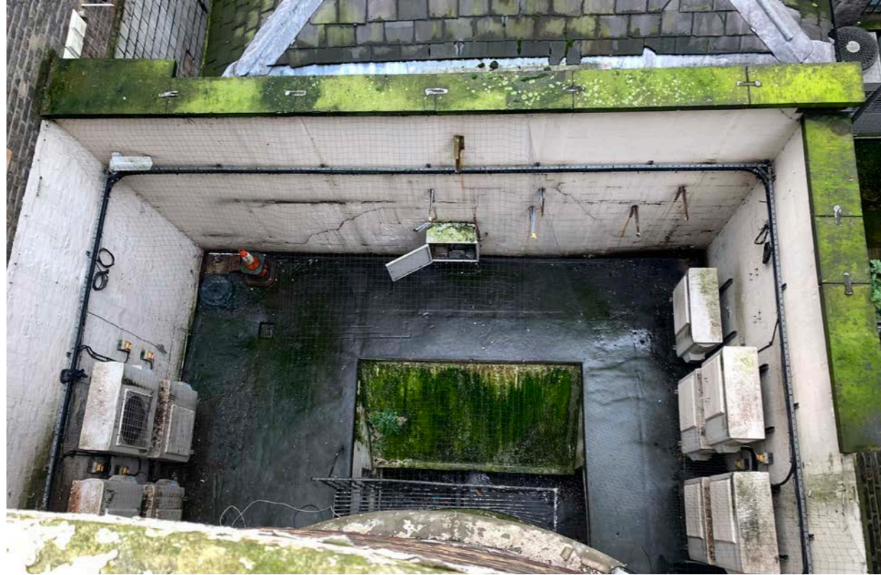
Figure 4. Rear of 22 Southampton Place.
