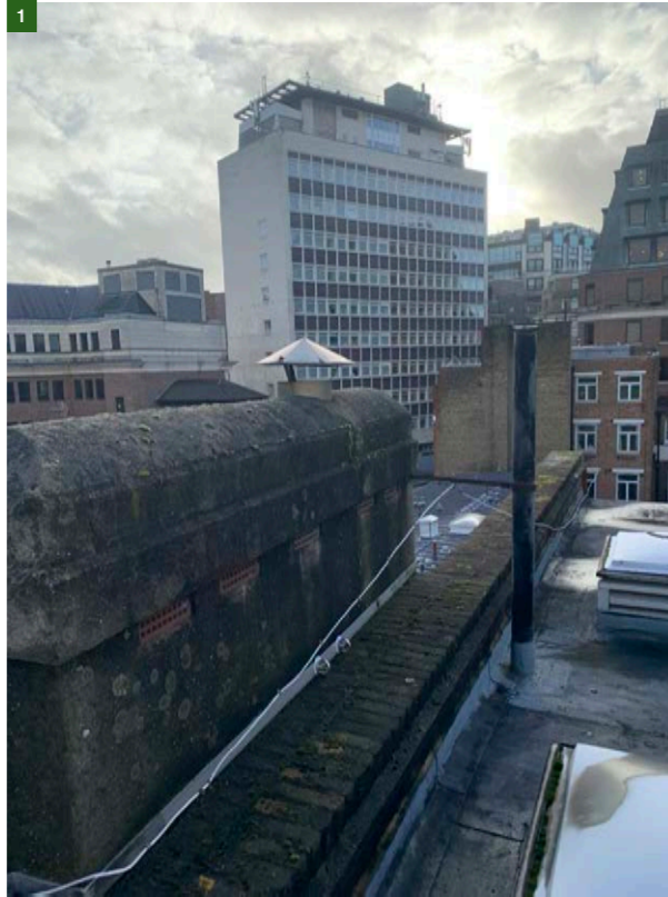
Figure 12. Existing capped chimneys.
