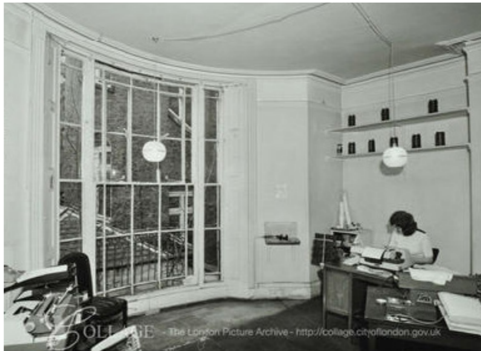
Figure 10. 22 Southampton Place, First Floor, Rear Room, c. 1971
