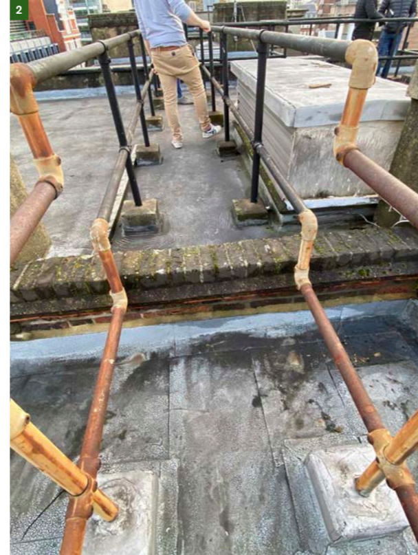
Figure 13. Access between 21 and 22 SP over party wall.
