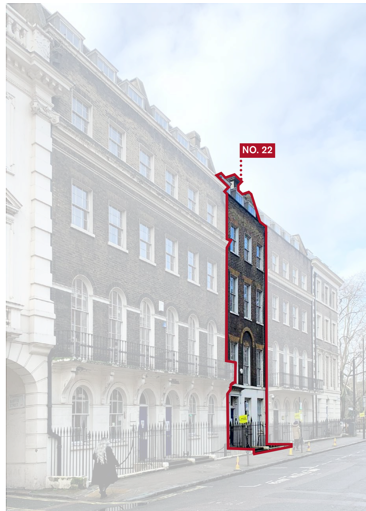
Figure 2. Frontage of No. 20 - 22 Southampton Pl.
