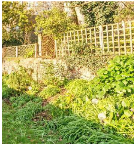
Existing garden wall with timber trellis is to be renovated.
