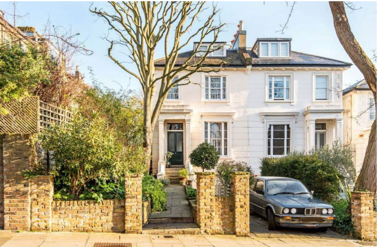
Existing front facade
