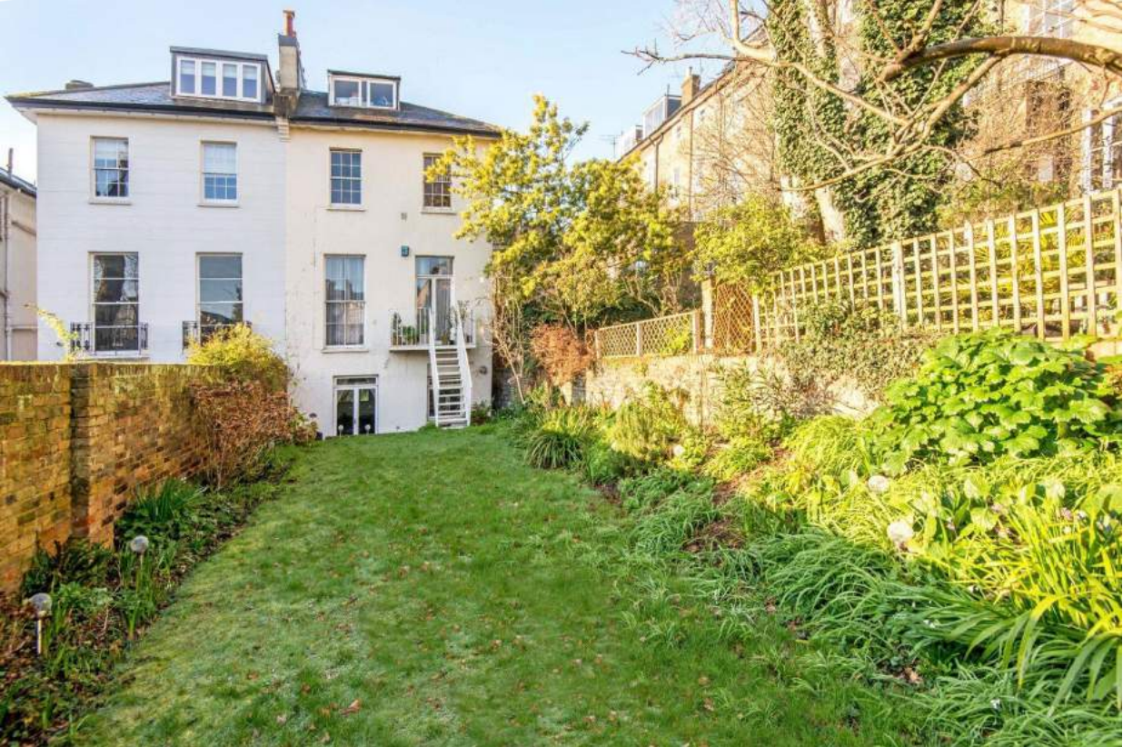
Existing rear facade
