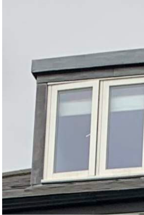
Lead clad dormer at No.19 Eton Villas
