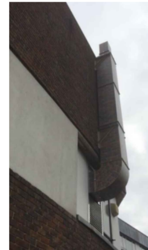
Photographic example of duct wrapped in brick effect vinyl. The brickwork graphic for this proposal will be printed to match the surrounding brickwork
