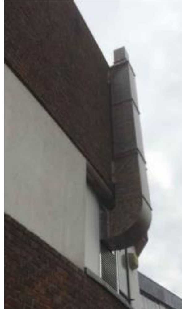
Left: Image of duct wrapped in brick effect vinyl
