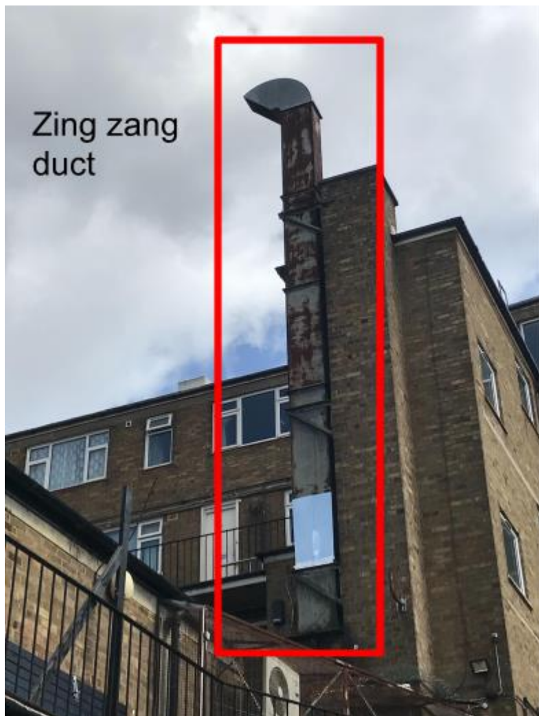
Above: Photo of the Z Zang extract duct at the rear of no. 115 Finchley Road
