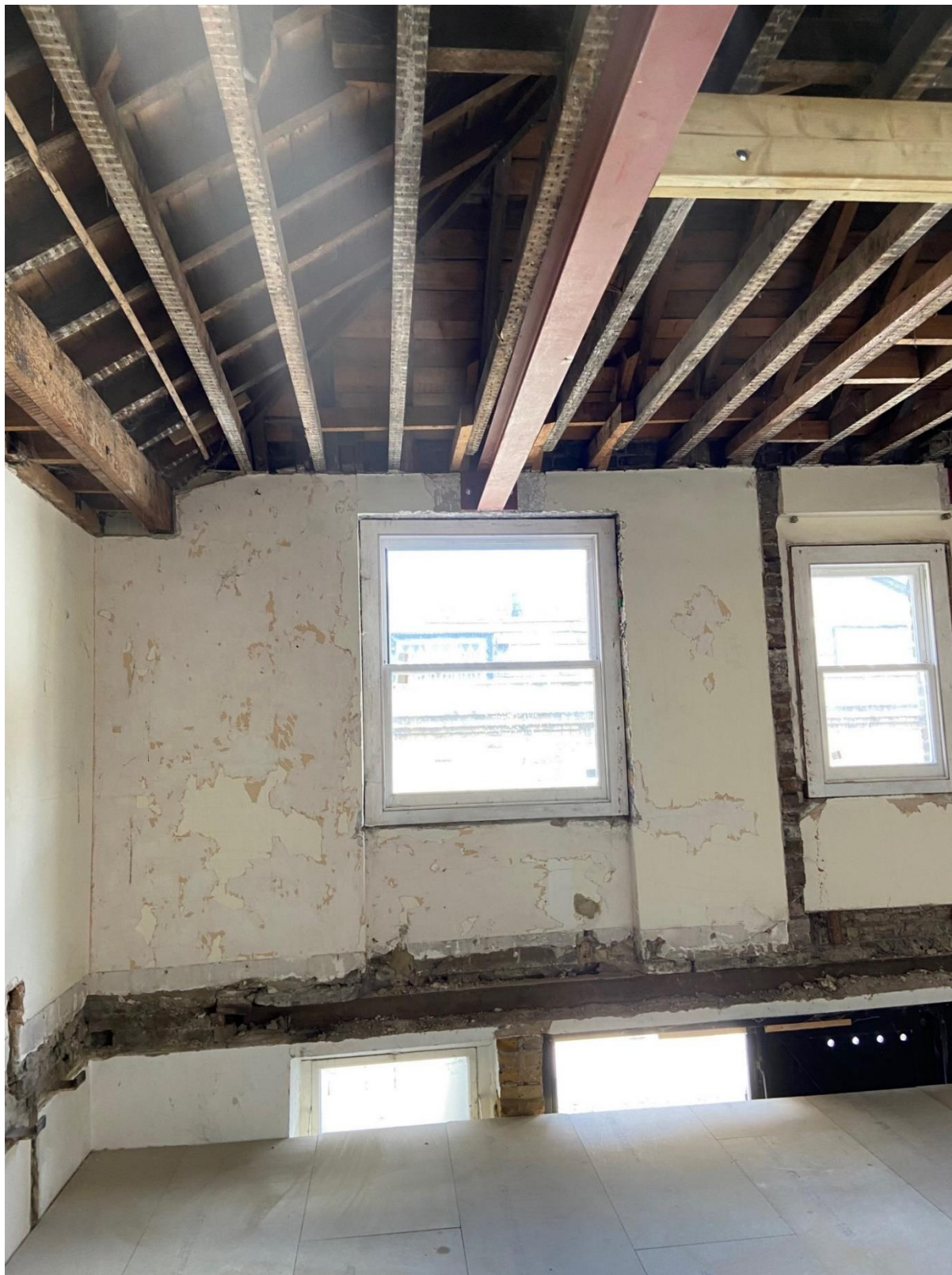
First floor ceiling beam north showing east end bearing
