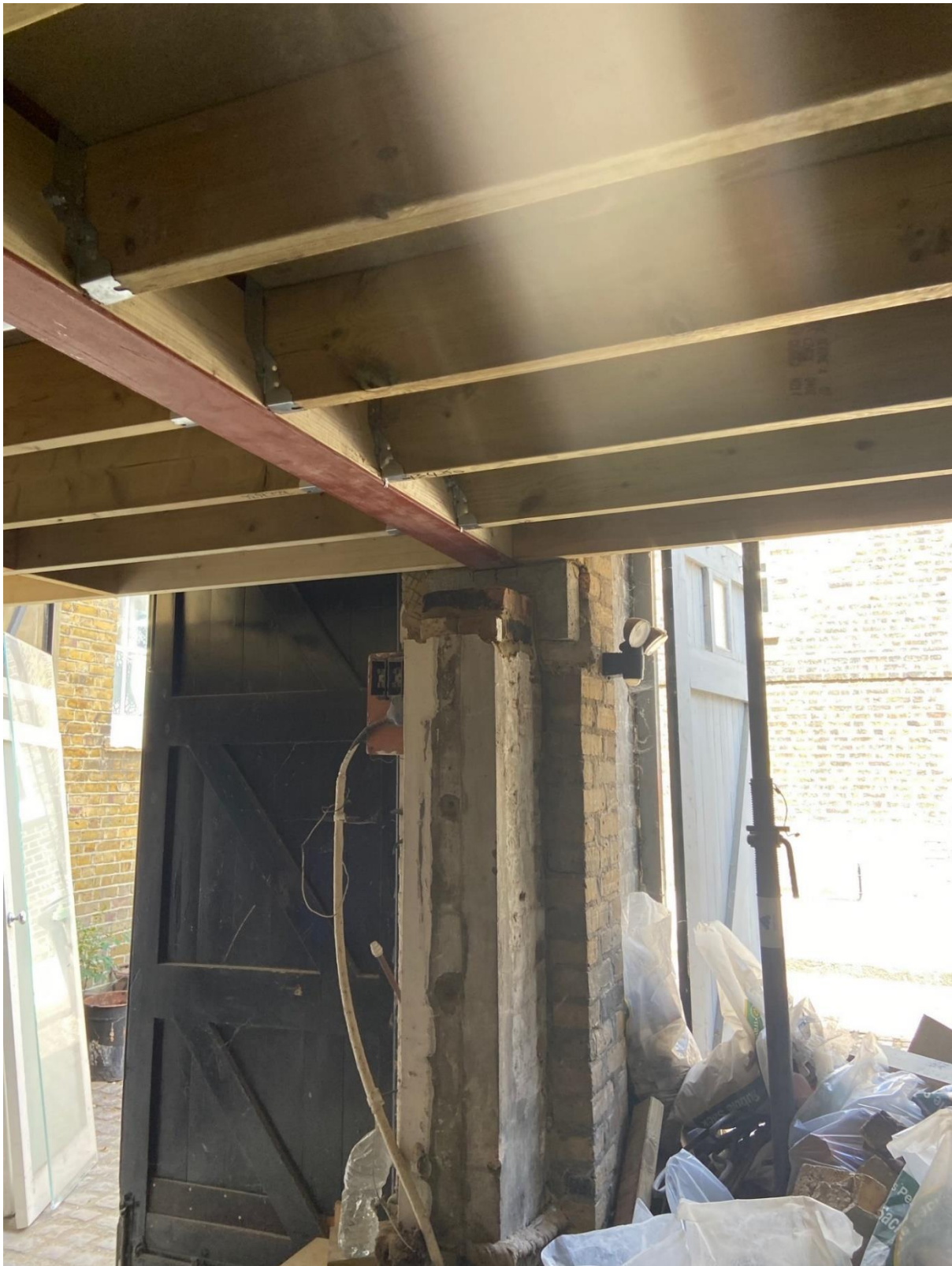
First floor timber joist bearing onto main beam south
