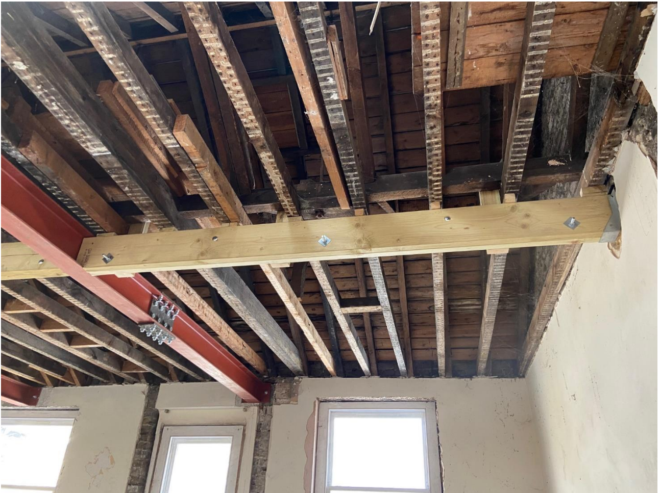
Ceiling beam central binder south end
