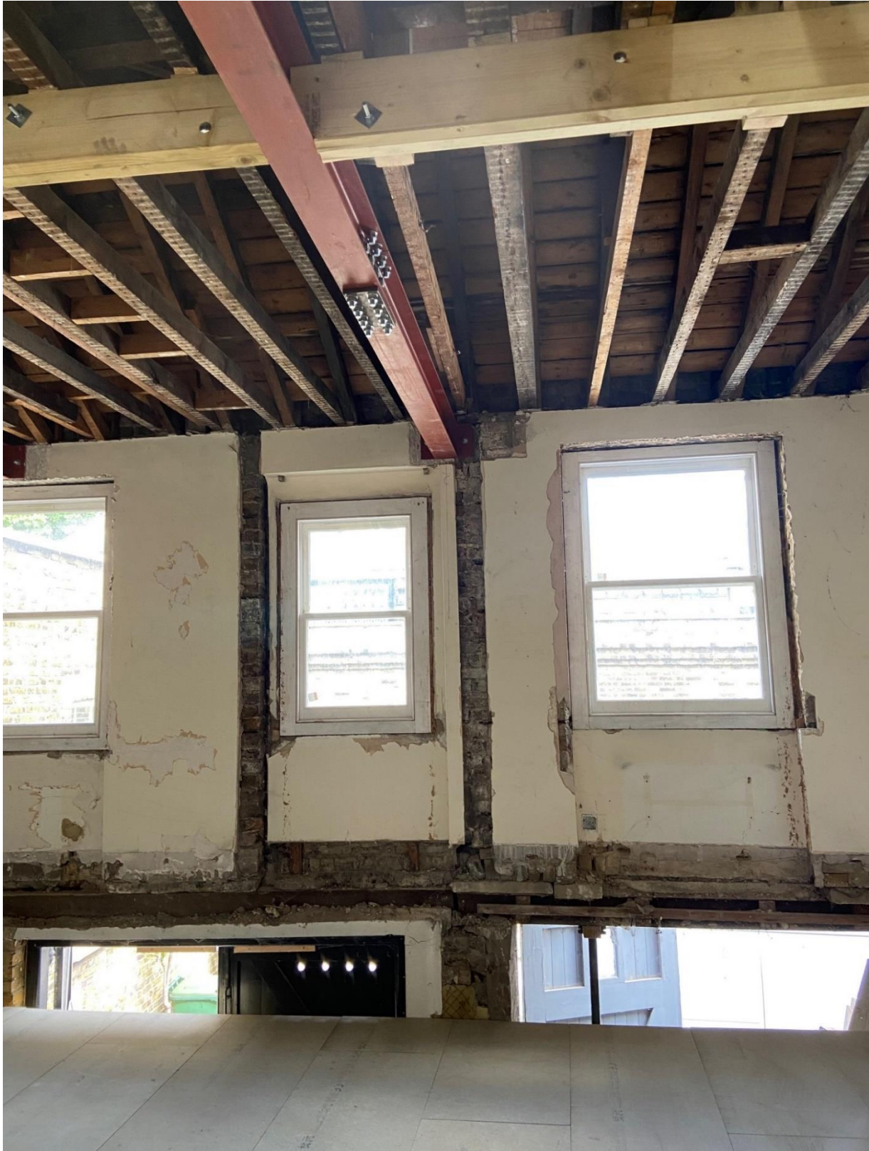
First floor ceiling beam south showing splice connection and east end bearing
