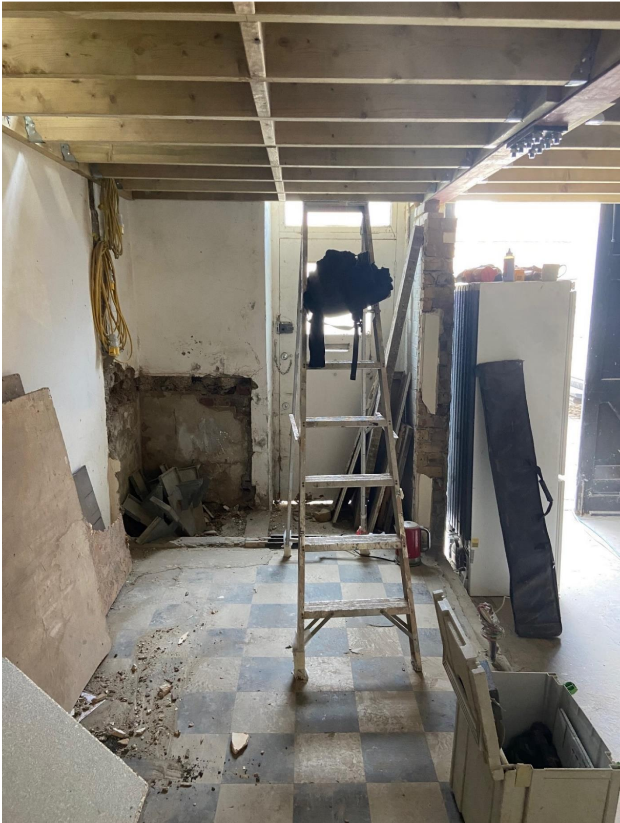
First floor blocking to joists
