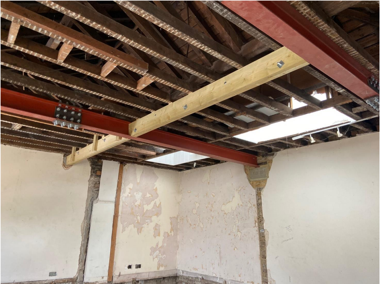
Ceiling beam central binder
