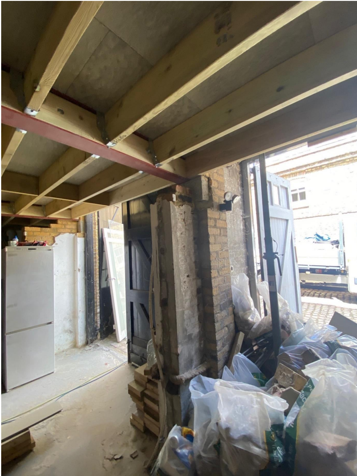
First floor main beam south, timber joist bearings
