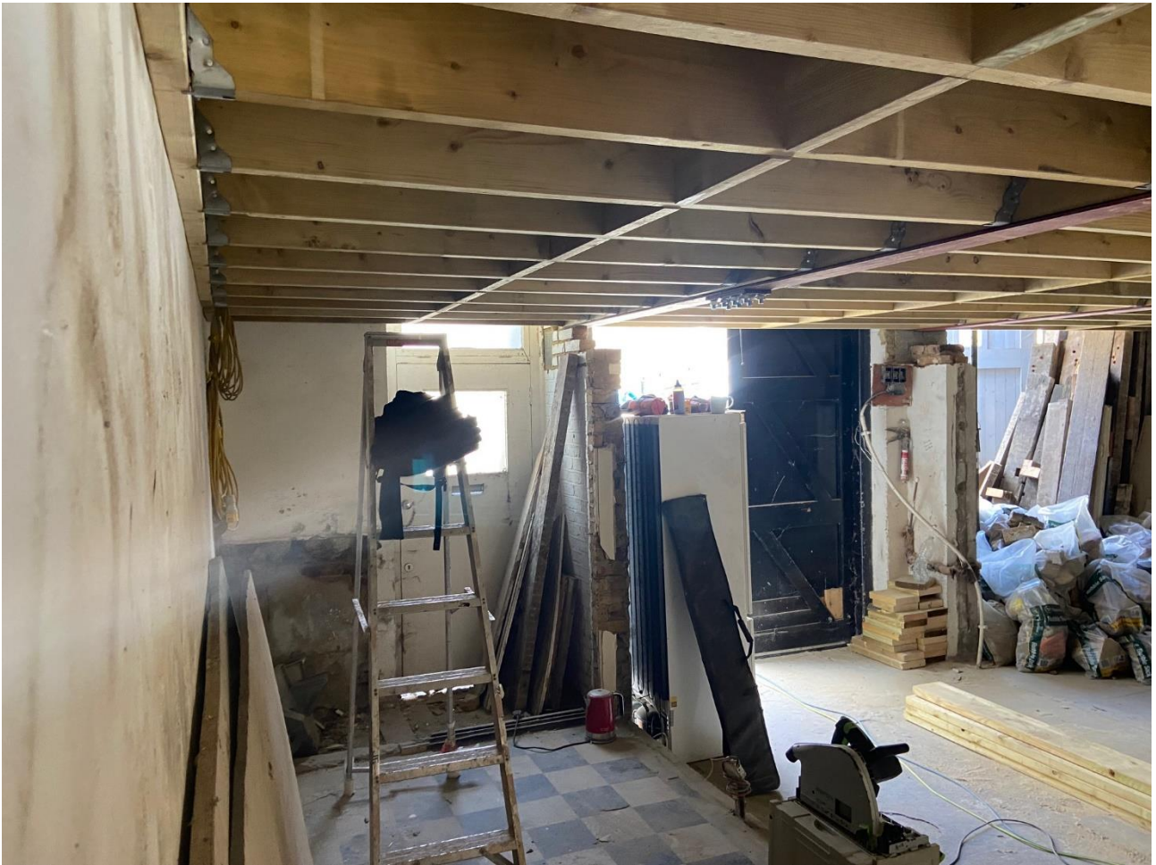
First floor, solid blocking to timber joists
