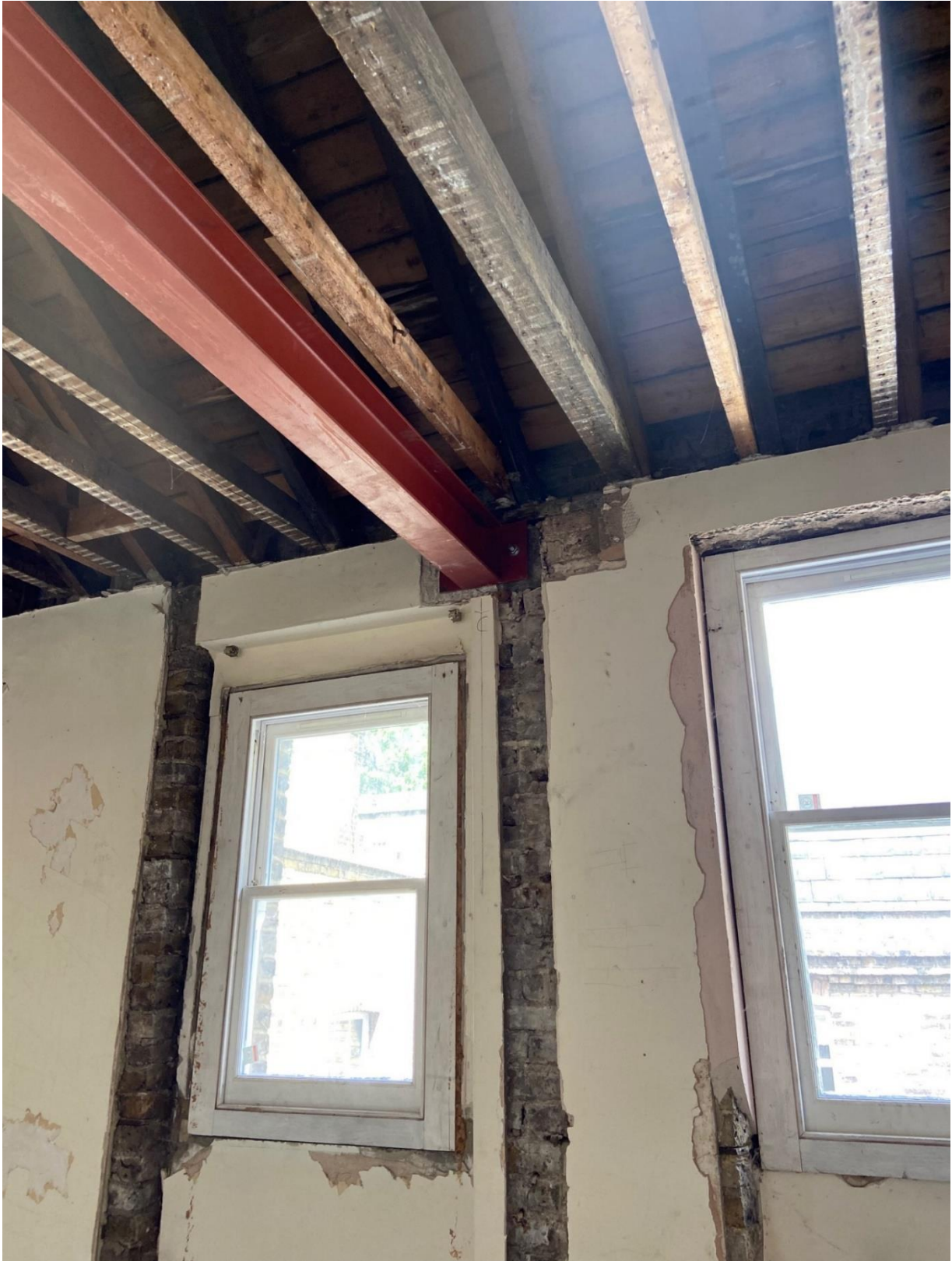
First floor ceiling beam south. East end bearing into existing brick pier
