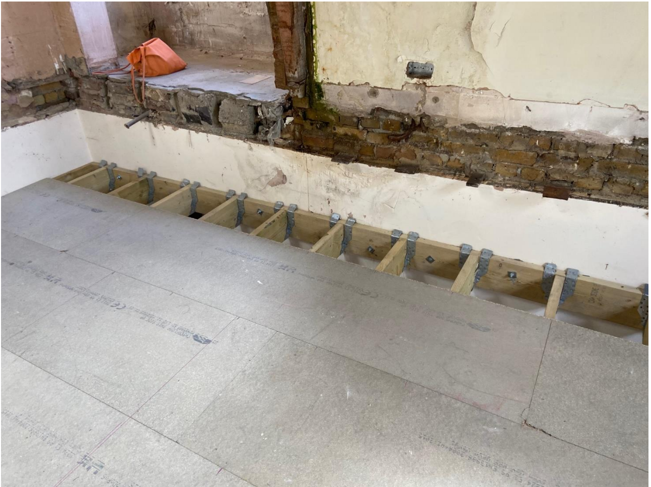
First floor, new floor north end bearing
