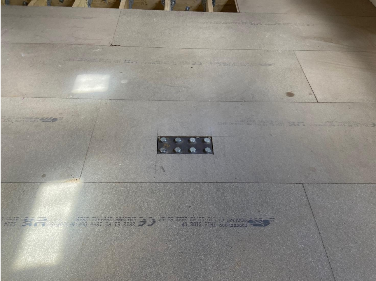
First floor, new floor main beam splice
