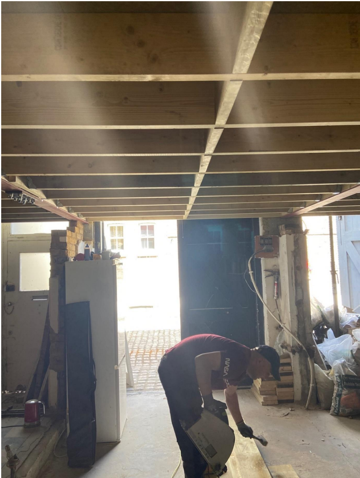
First floor timber blocking to joists
