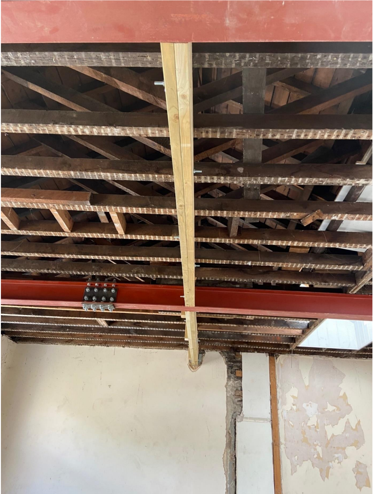
Ceiling beams, central binder
