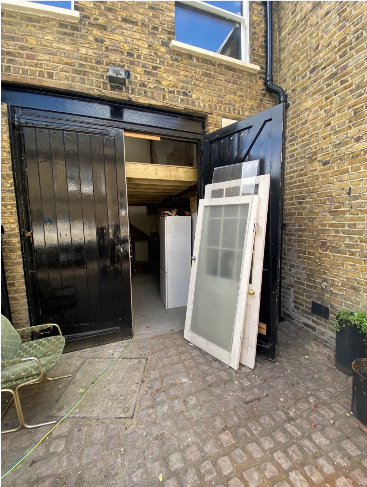
Entrance door, existing lintel retained. Mews house, part of 12 Gloucester Gate
