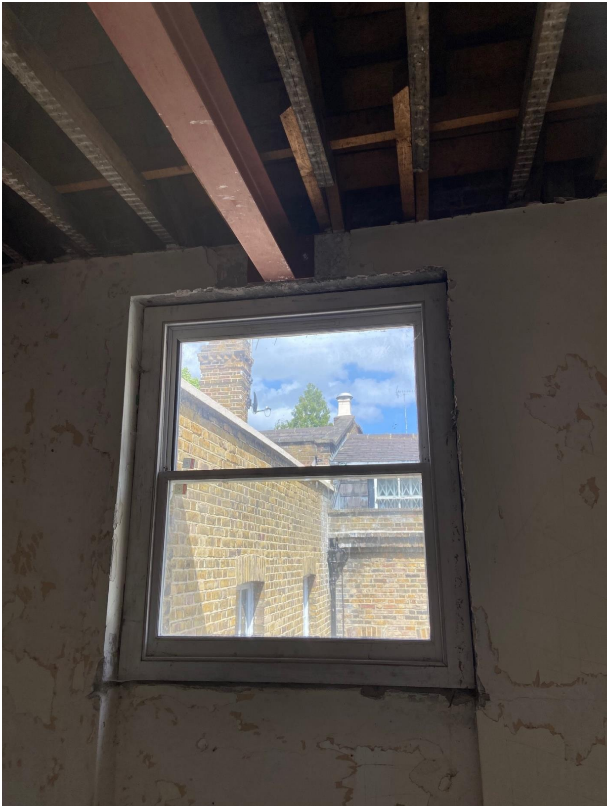
First floor ceiling beam north. East end bearing into existing window lintel
