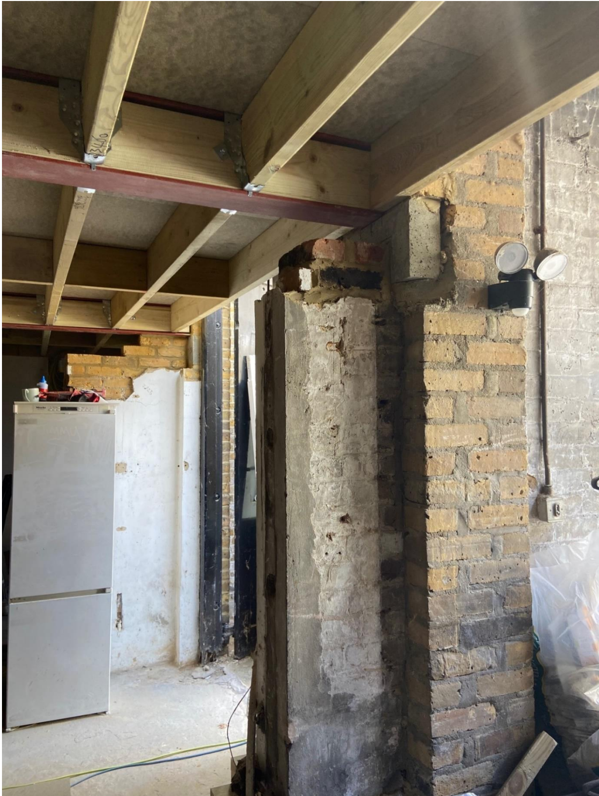
First floor main beam south, east end bearing
