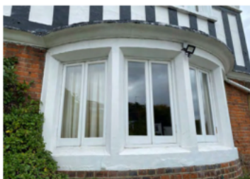
Example of identical bay at Old Hall
