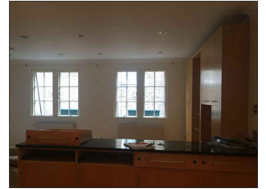
Existing 1st floor dormer windows
