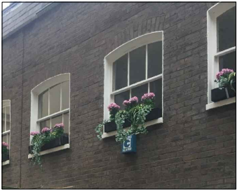
New Sash Windows Traditional sliding box sash. Double glazed white painted timber with glazing bar to match existing.
