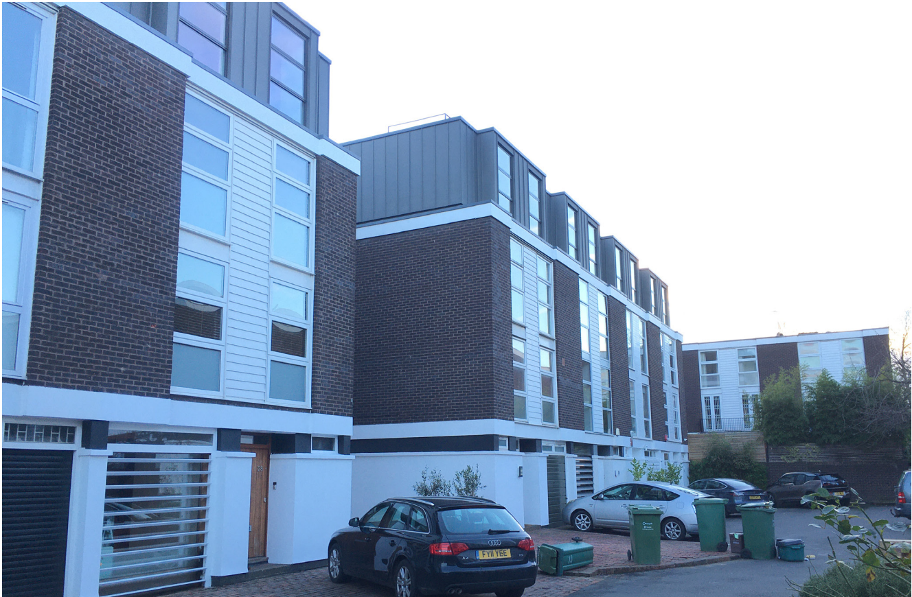
Roof extensions to 24-34 Elliott Square, view from Elliott Square
