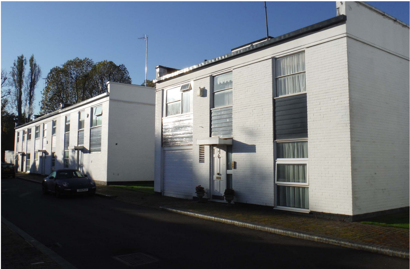
View of typical 2 storey houses in Quickwood
