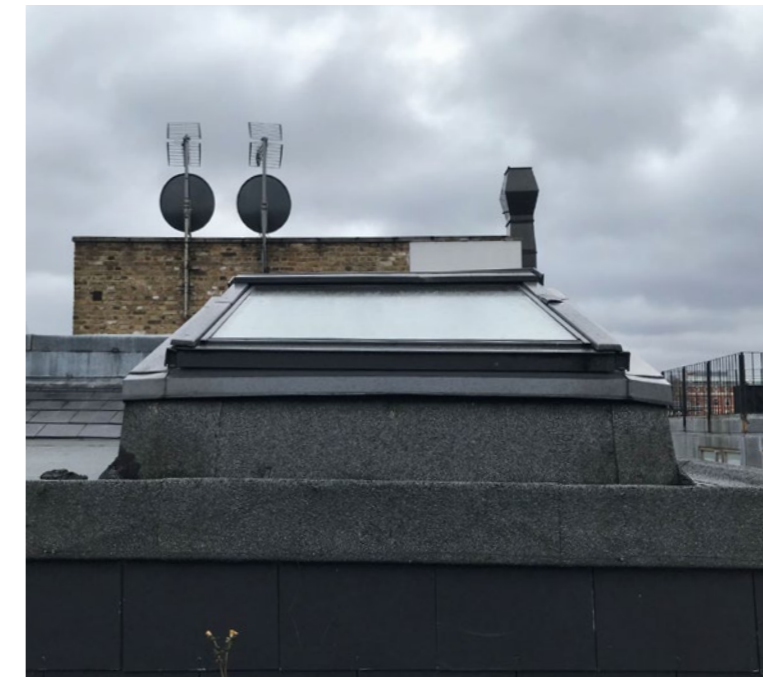
No. 197 neighbouring skylight
