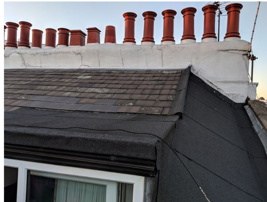
Roofing felt dormer and chimney stacks
