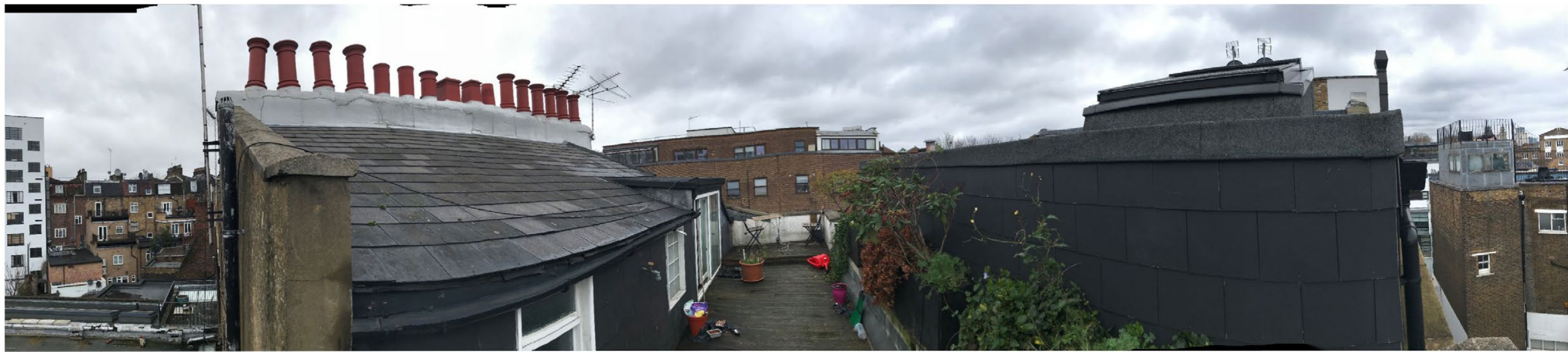
View onto 201a roof terrace
