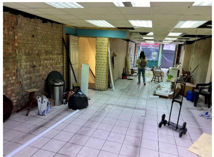
Existing front of shop/access to basement
