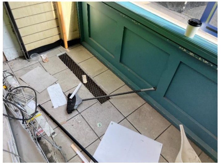
Existing vent from basement
