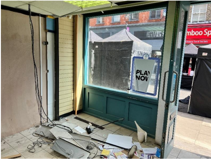
Existing Internal shop front
