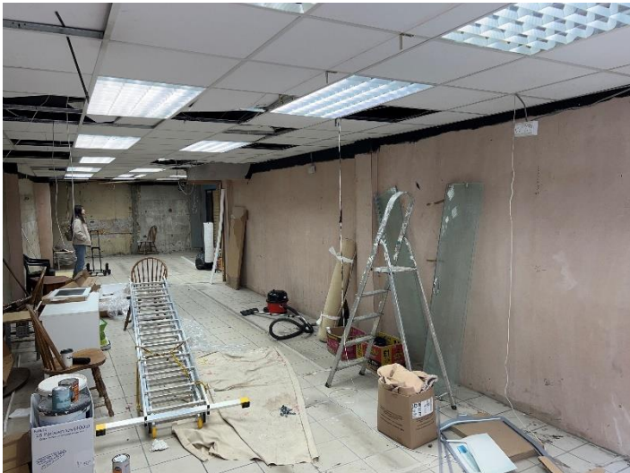
Existing Internal shop front
