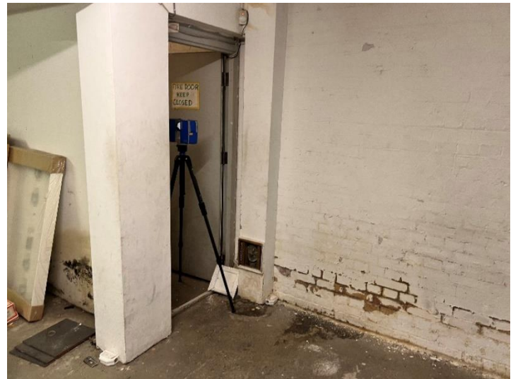
Basement entrance door
