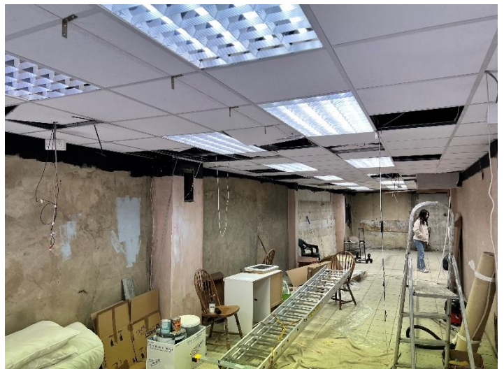
Existing vent from basement
