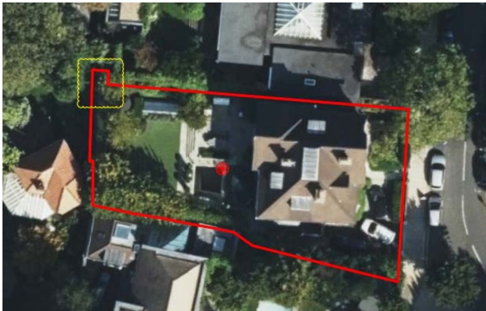
Figure 1: Site location shown on AutoCAD geolocation satellite image; yellow cloud identifies area of re-development
