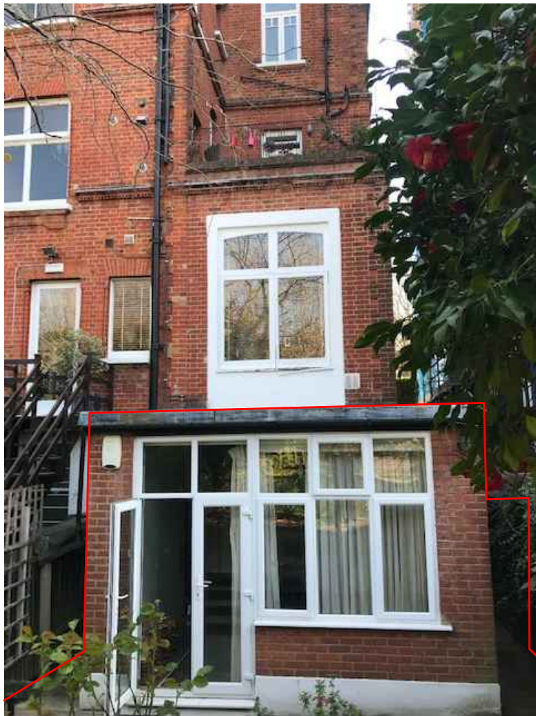
Existing Rear Extension
