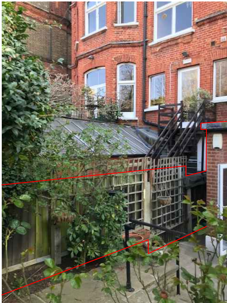
View towards existing neighbouring extension
