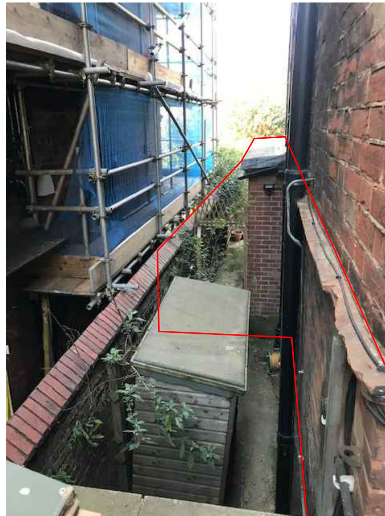
View from the front side elevation
