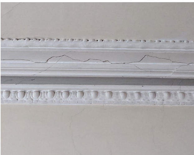
Fig. 3 Typical example of the existing condition of the cornice on the raised ground floor showing cracking in the top section and an in-tact section below.
