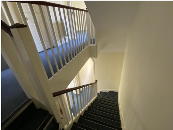
Figure 30: The modern secondary staircase.
