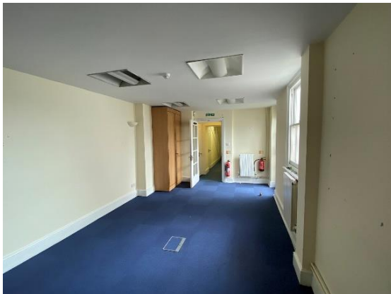
Figure 24: The basement room within the part width rear addition looking back towards the house.
