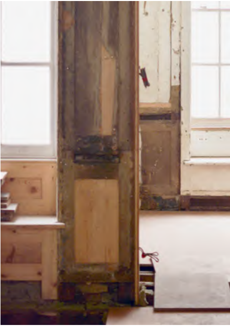
Restoration of wall paneling at 34 Great James Street with piecing in where required
