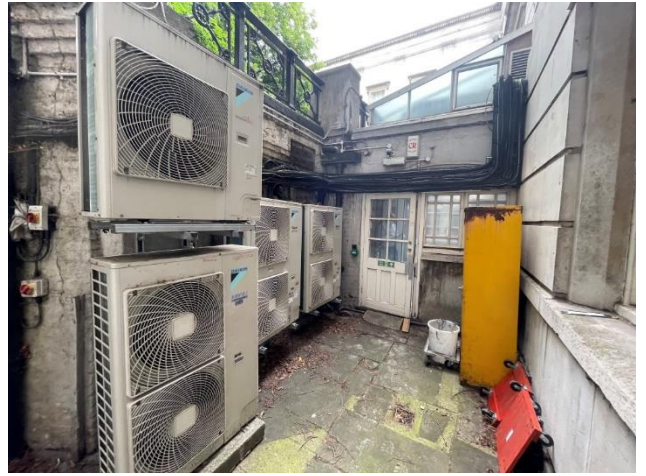
Entrance to well from shop
