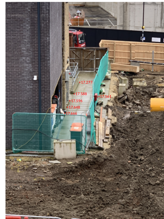
Image showing existing Calthorpe House Bin Store & Access (bin store and access ramp retaining wall to be retained)
