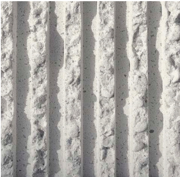
C3 - Concrete columns Material: White precast concrete (Reckli formwork) Supplier: Chiltern GRC Finish: Acid Etched
