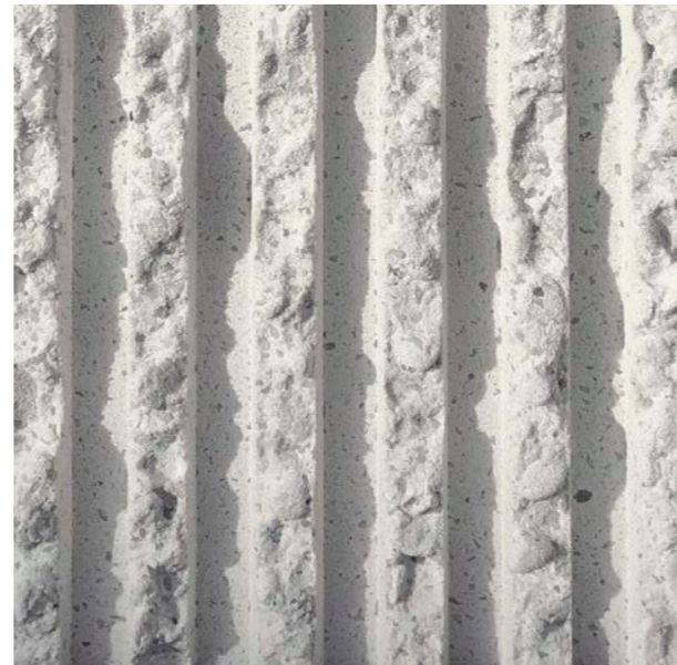
C3 - Concrete columns Material: White precast concrete (Reckli formwork) Supplier: Decomo Finish: Acid Etched
