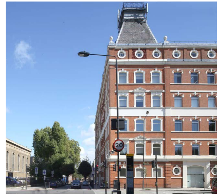
The Centro Building, 100m west of the site
