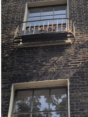
Iron balustrade (this one at 2 nd floor level)
