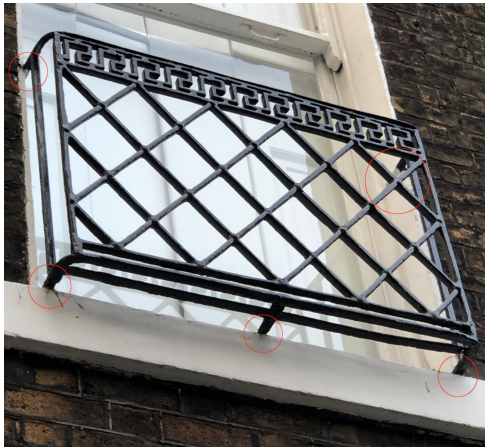
Original iron balustrade fixtures
