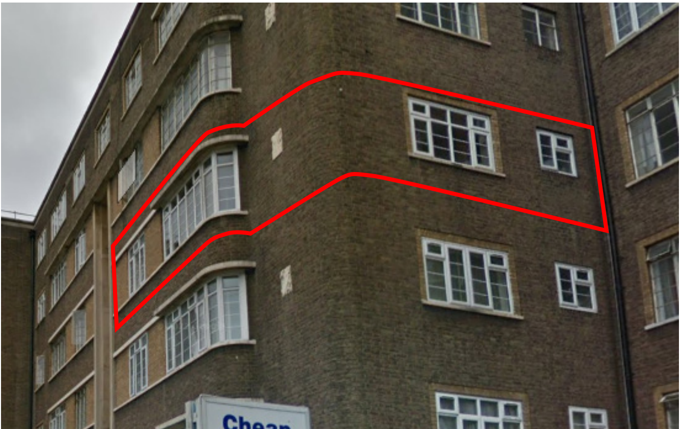
Above: Replacement uPVC windows as seen from Avenue Road, May 2014. Source: Historic Google Streetview
