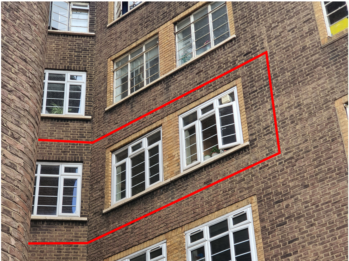
Above: Flat No. 81, courtyard-facing elevation
