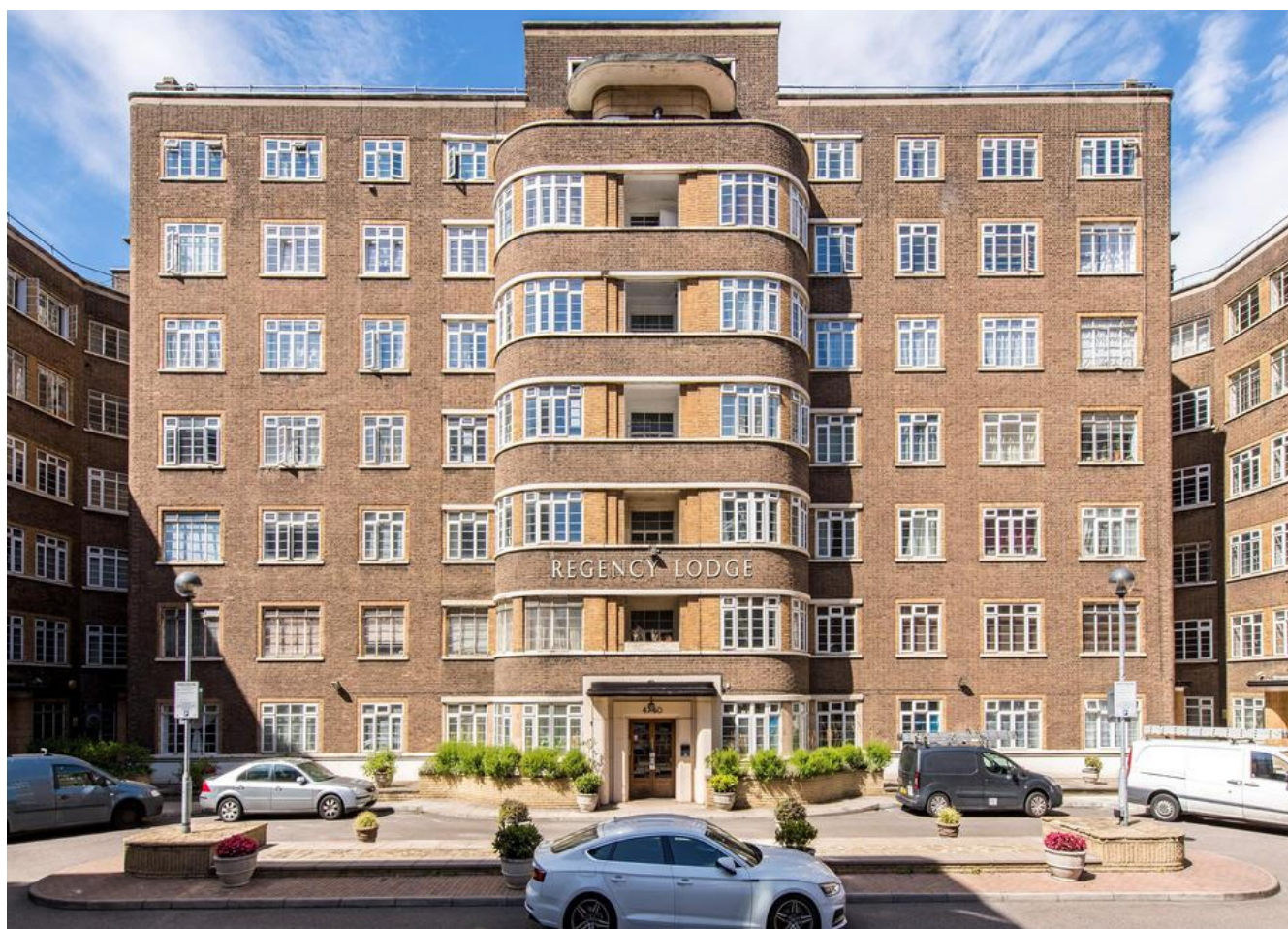
Above: Regency Lodge, main entrance
