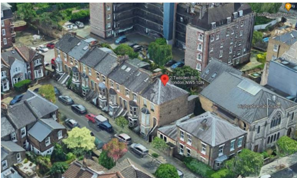
Aerial views showing hipped roofs in area
