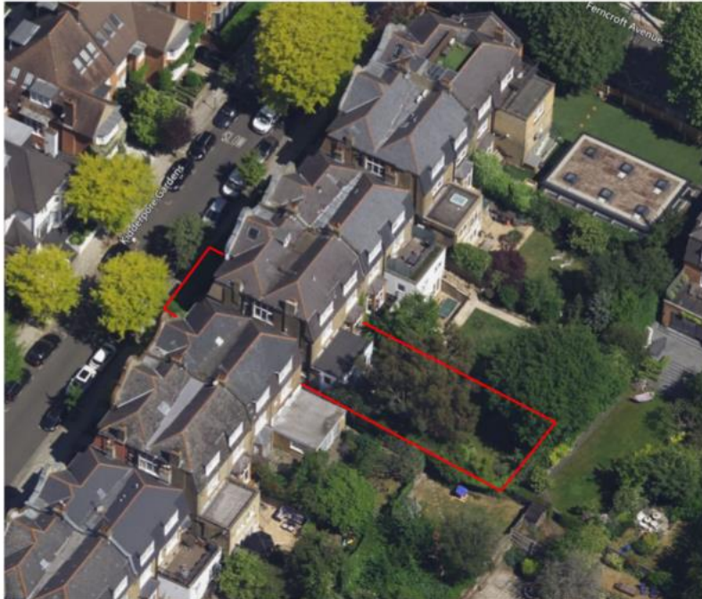
1. Aerial view with site in red
