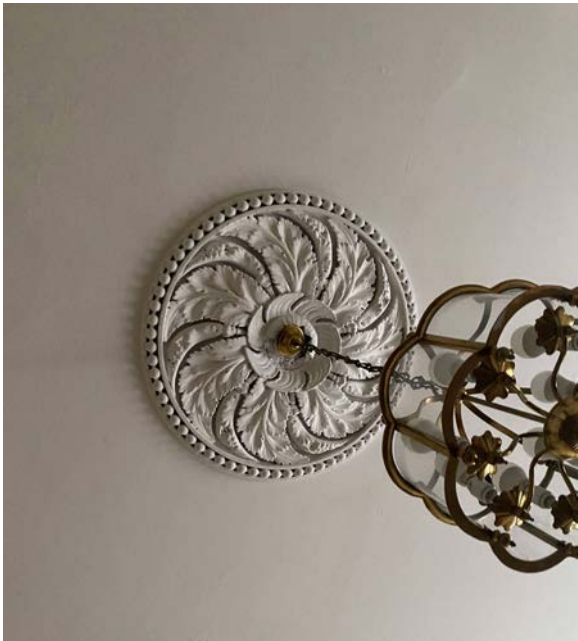
Existing ceiling rose in No. 7. All ceiling roses to be re-used with new pendant light fitting
