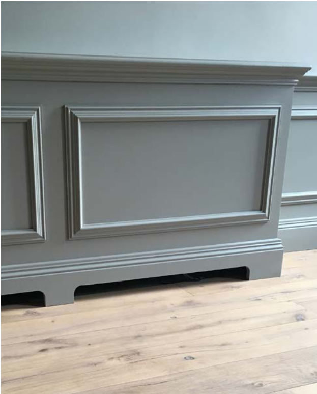
Example of wall casing to conceal VRF unit
